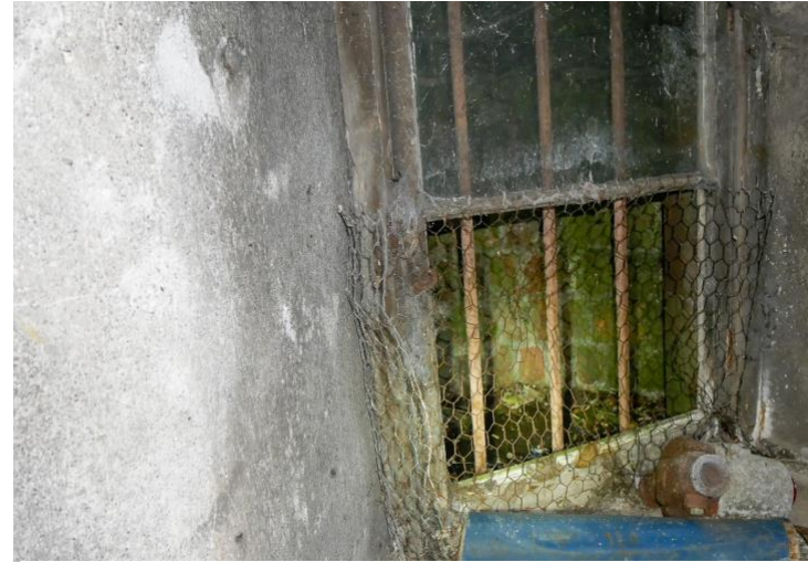
3. Fine chicken wire mesh on access to cellar from external opening. This opening has been sealed shut
