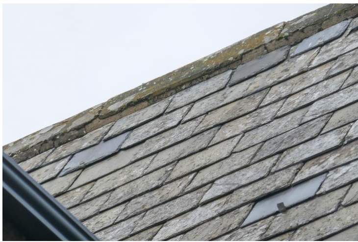
1. Example of roof and ridge tiles. Existing roof will be retained on most of the building apart from the areas to be removed. So ridge and roof tiles will be repaired, repositioned or replaces where necessary
