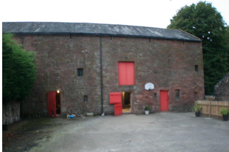
Barn & yard from the east
