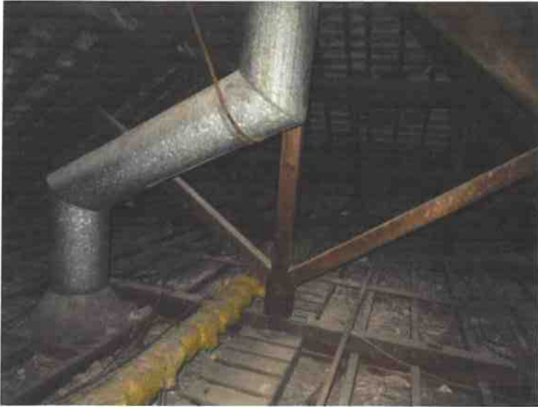
Photograph 27 – Loft spaces Lofts 2 and 5 are both of king post construction.
