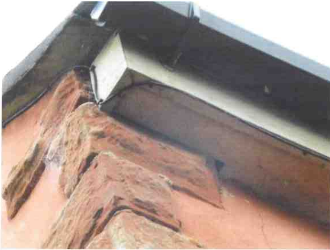
Photograph 9 – Gap between boxed soffit and wall on the western aspect of the extension.
