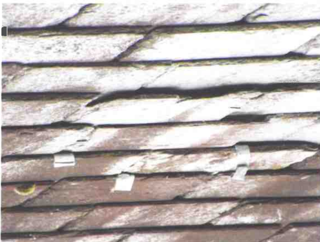
Photograph 17 – Raised roof tiles on the western aspect of the hotel.
