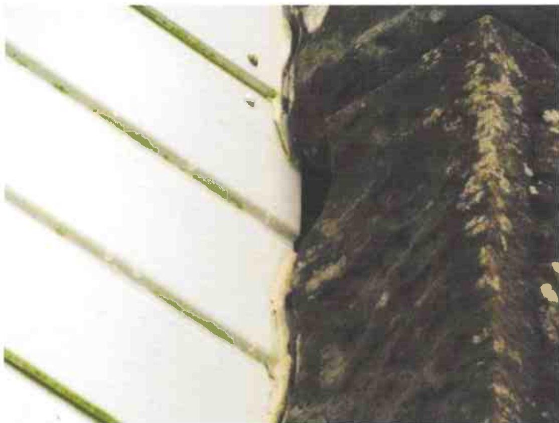
Photograph 15 – More gaps between stonework and window, same location as Photograph 14.
