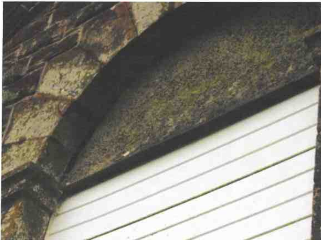
Photograph 14 – Gaps between stonework and window arch on the southern aspect of the hotel.
