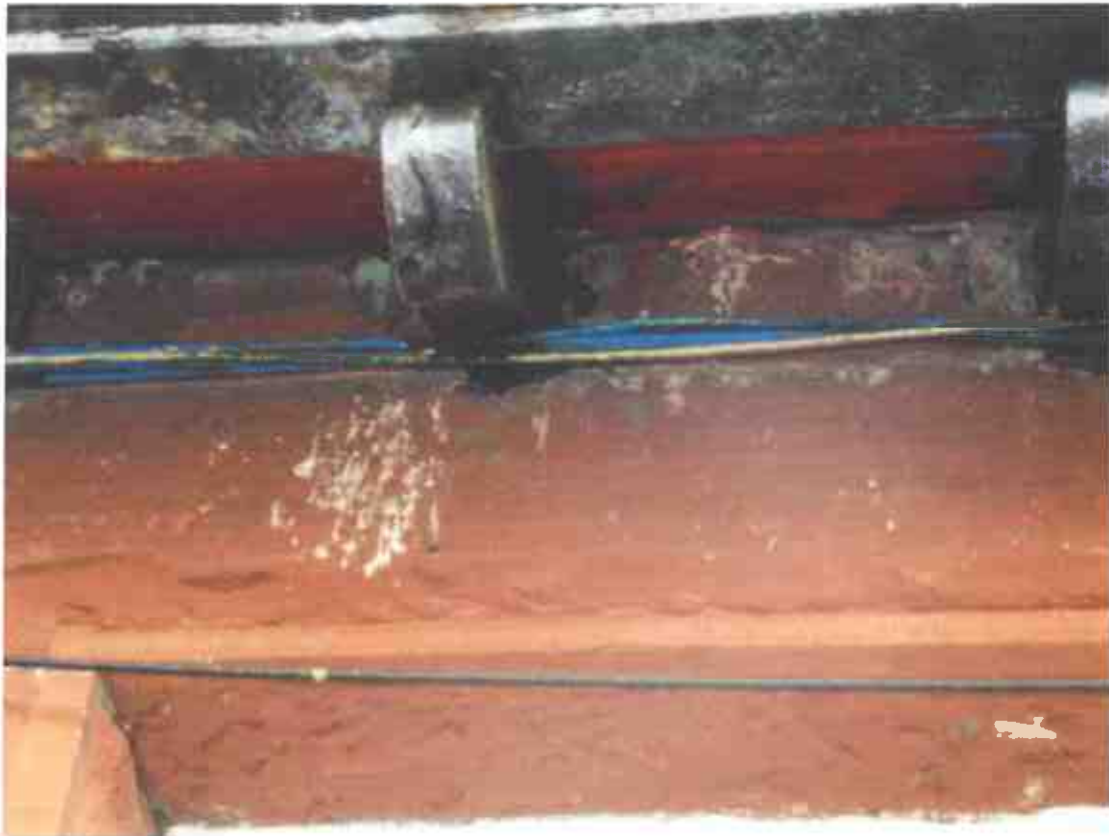
Photograph 21 – Evidence of bird activity under the wooden eaves on the northern aspect of the hotel.
