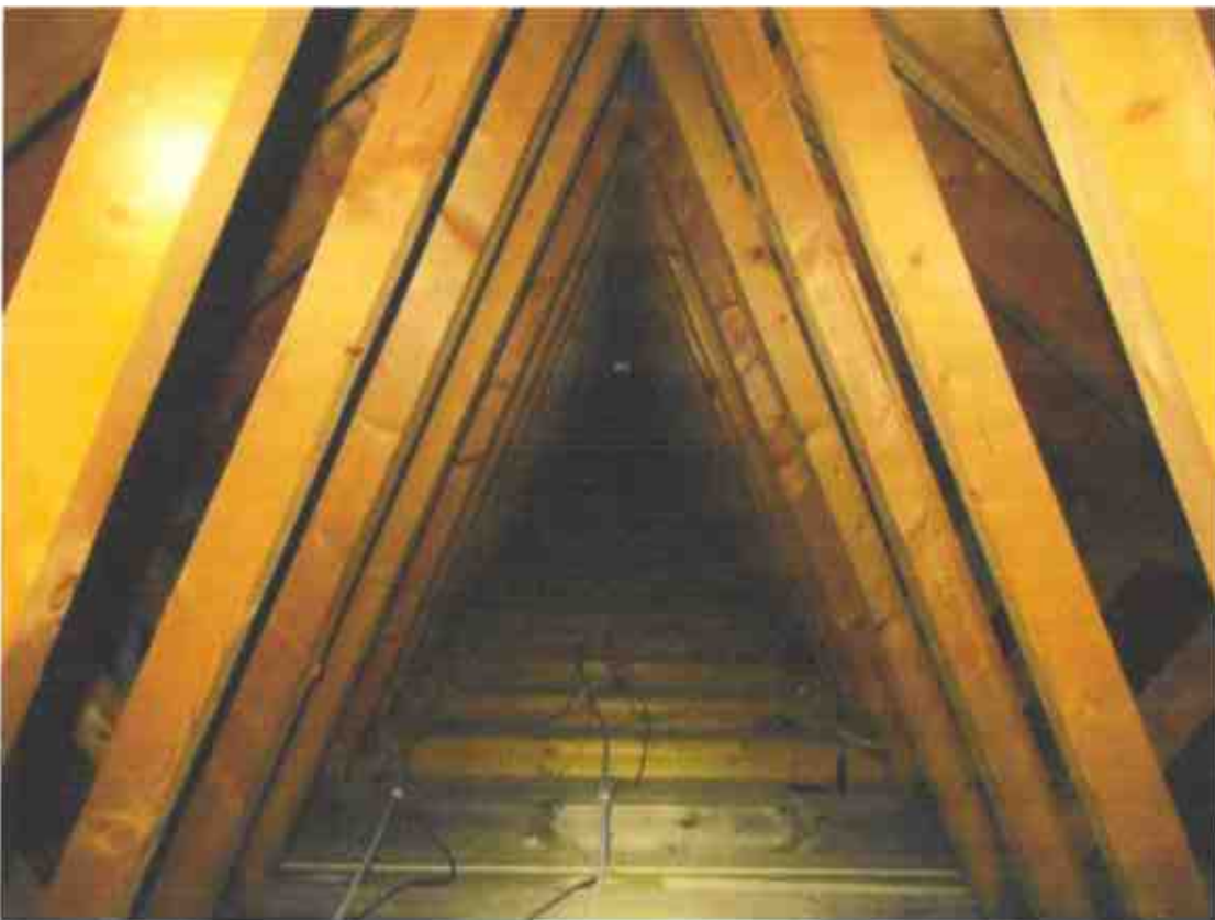
Photograph 24 – Loft space within the extension (Loft 1) is of a trussed construction.
