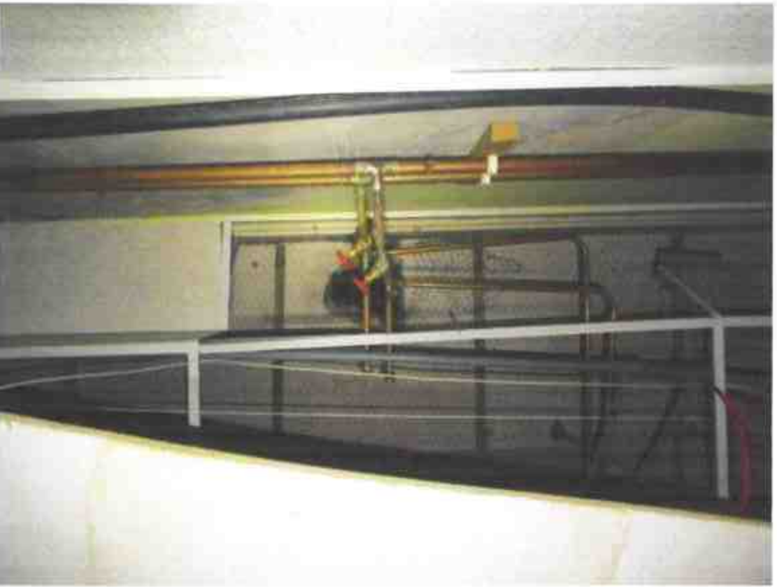
Photograph 29 -- At least three layers of false ceiling that leads to Loft 6.
