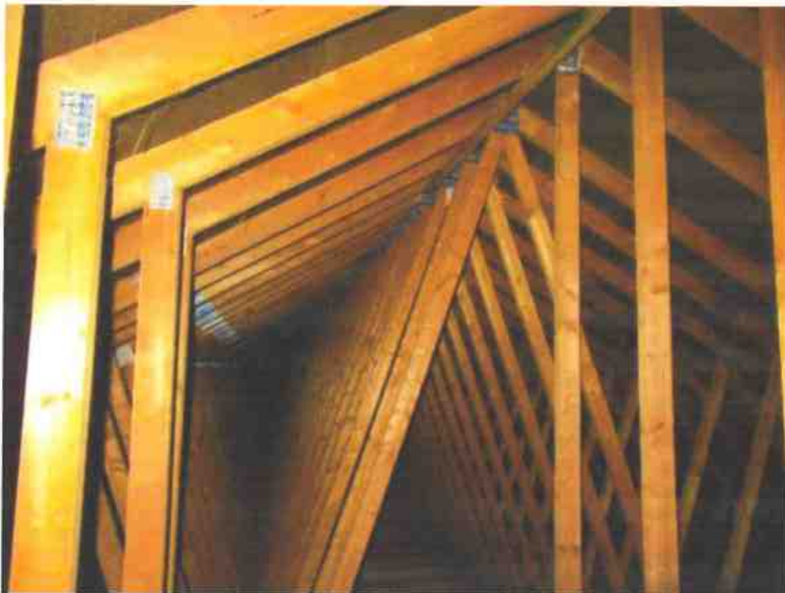
Photograph 26 – Loft space within the main section of the old build (Loft 3) is of trussed construction.
