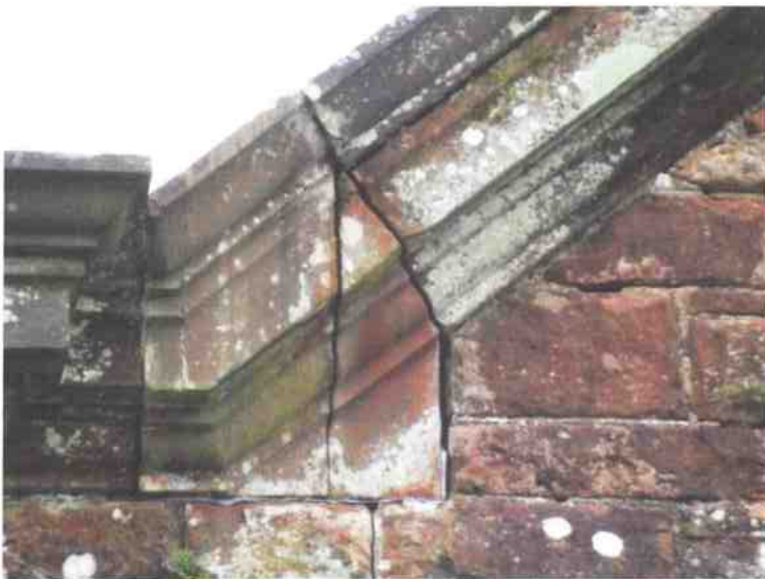
Photograph 16 – Gaps at the coping stones on the southern aspect above the conservatory.
