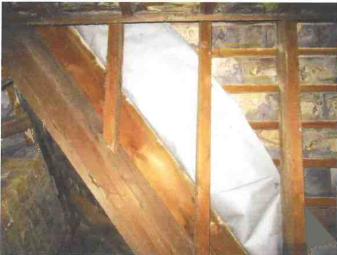
Photograph 28 – A small section of Loft 5 is lined with breathable membrane.
