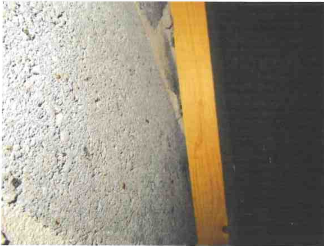
Photograph 25 – Gaps between the beams and wall at each gable ends of the extension.
