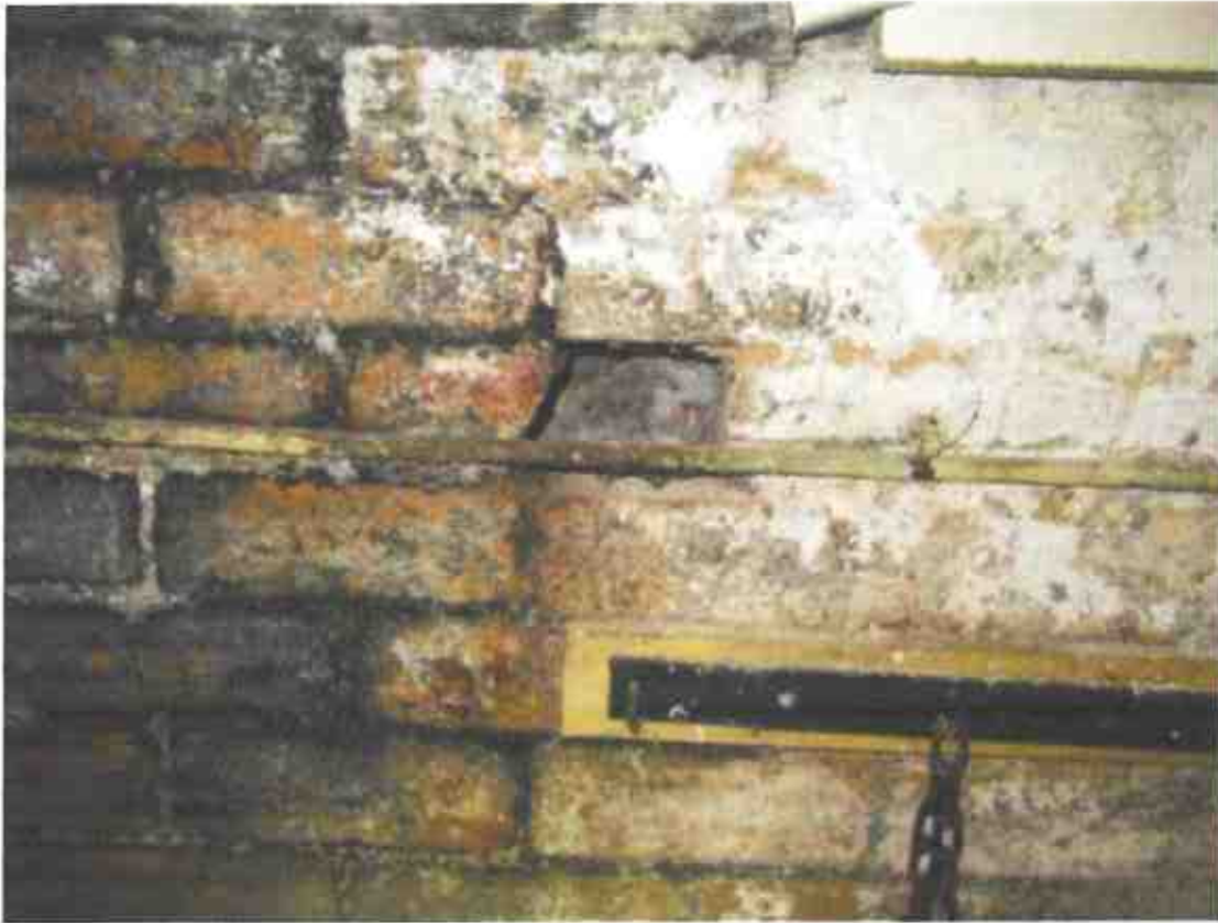
Photograph 31 – Gap into the wall cavity of the cellar.
