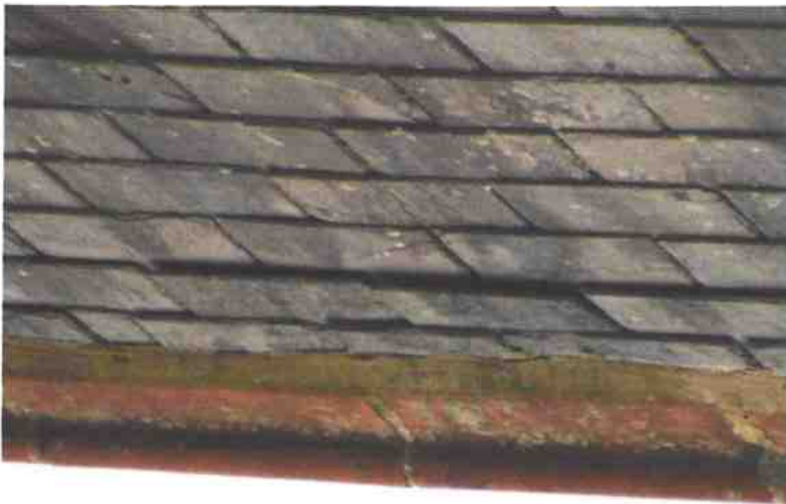
Photograph 18 – Raised roof tiles on the northern aspect of the hotel.
