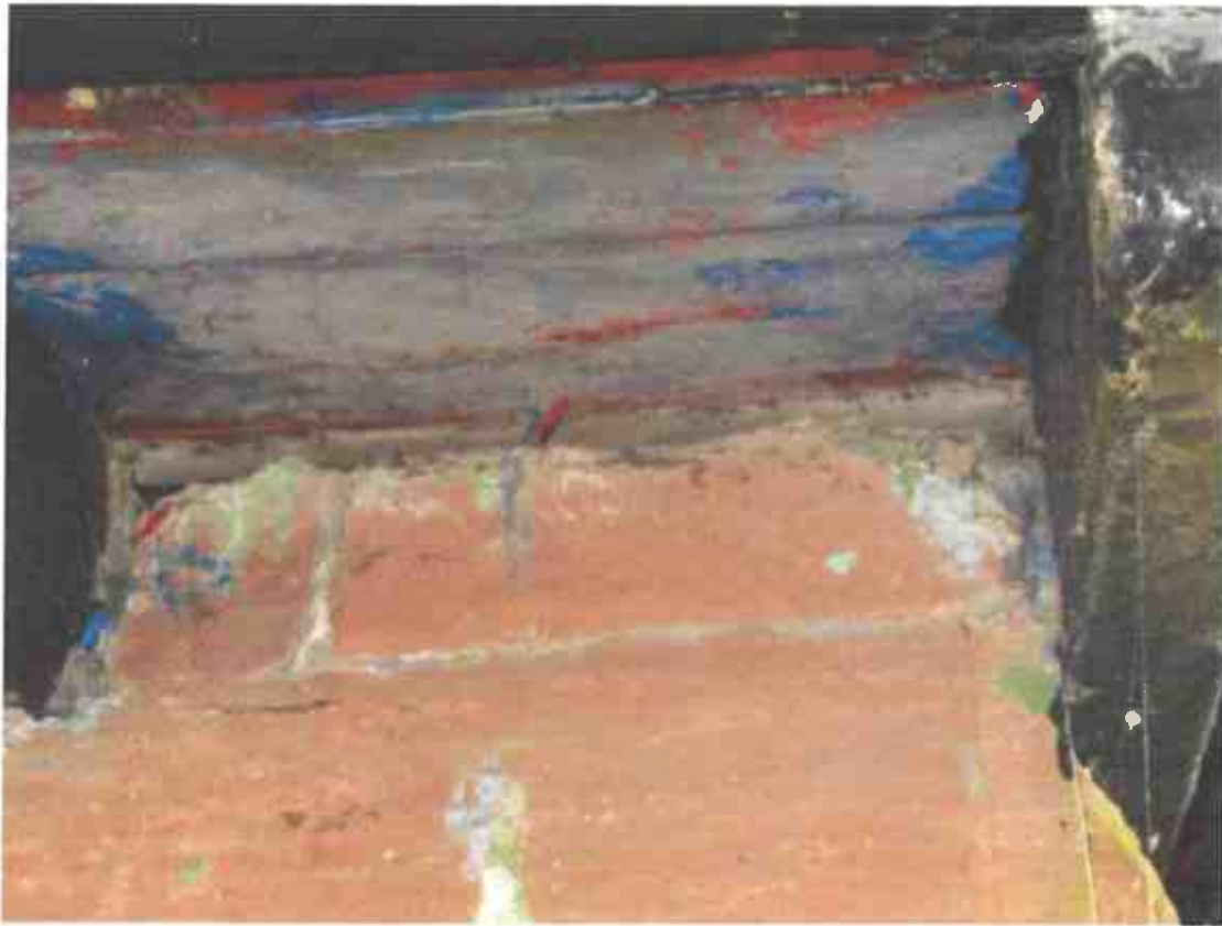
Photograph 19 – Gaps under the wooden eaves on the northern aspect of the hotel.
