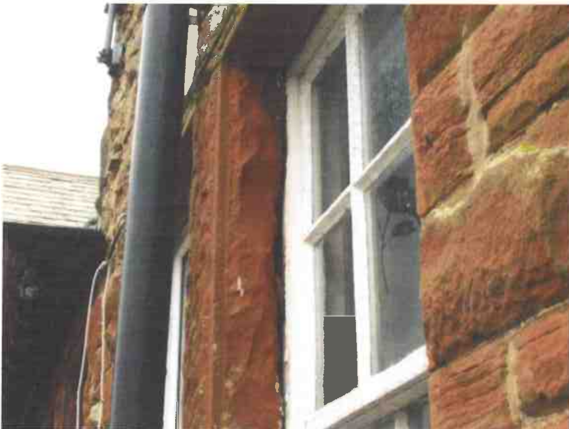
Photograph 20 – Gap between the stonework and wooden window on the northern aspect of the hotel.
