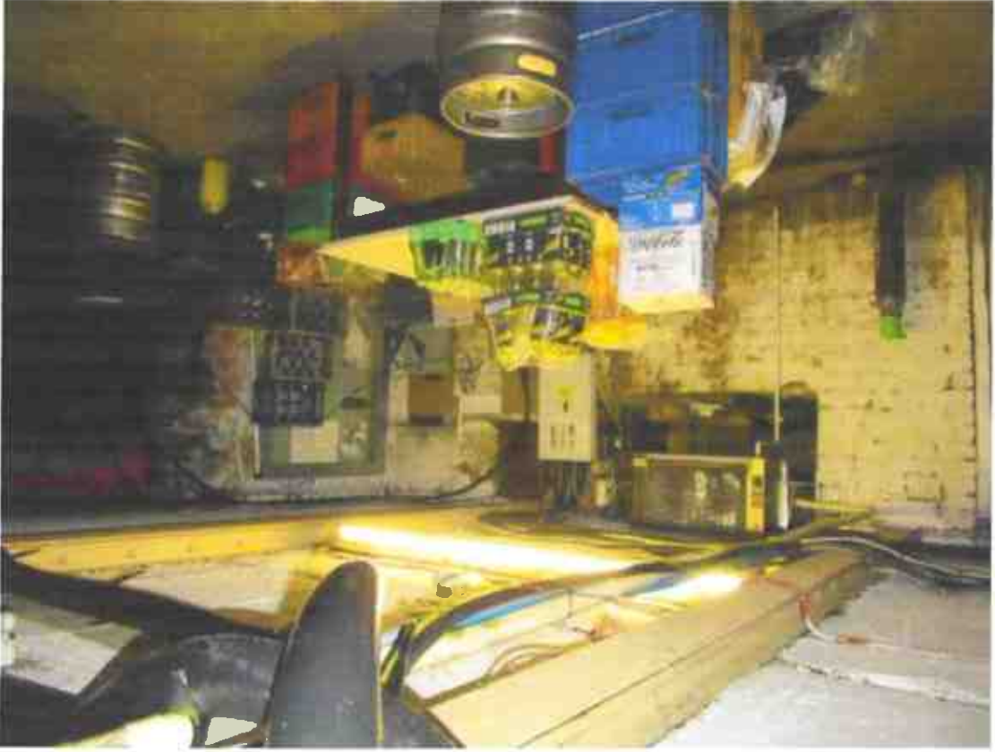
Photograph 29 -- At least three layers of false ceiling that leads to Loft 6.
