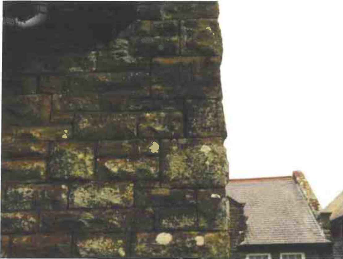
Photograph 13 – Gaps in the stonework on the southern aspect of the hotel.
