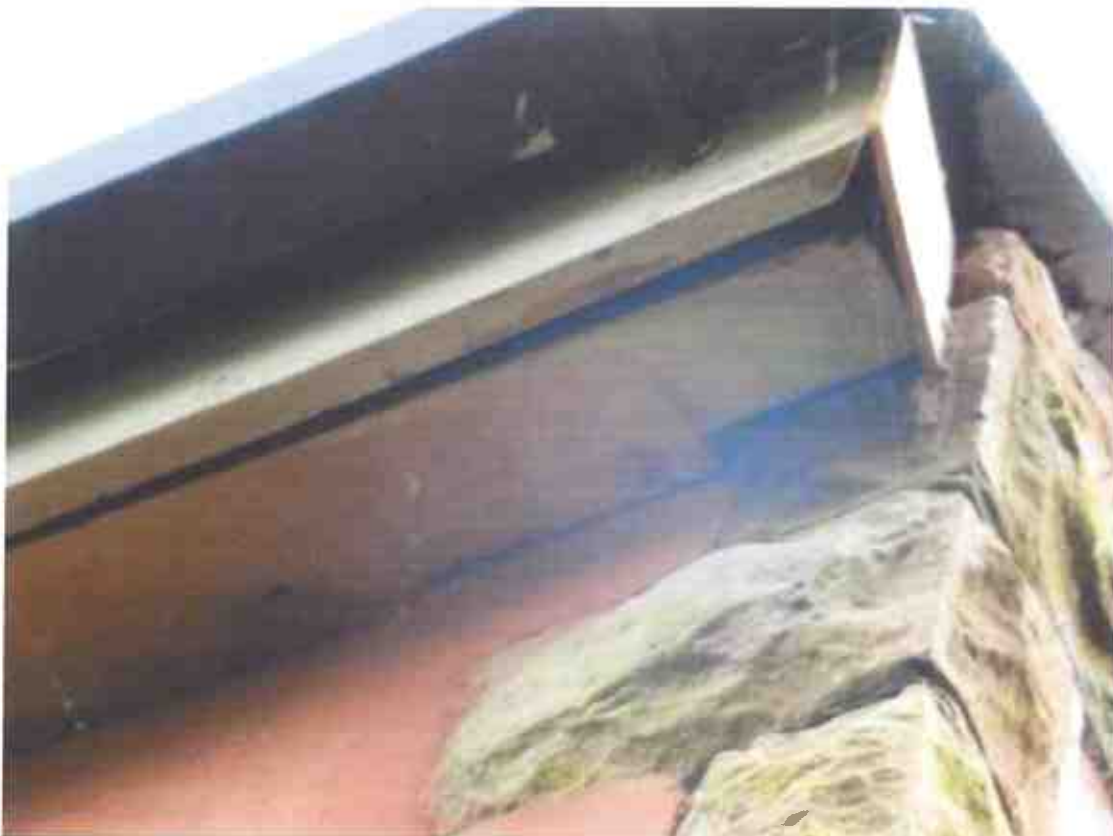
Photograph 10 -- Gap between boxed soffit and wall on the eastern aspect of the extension.
