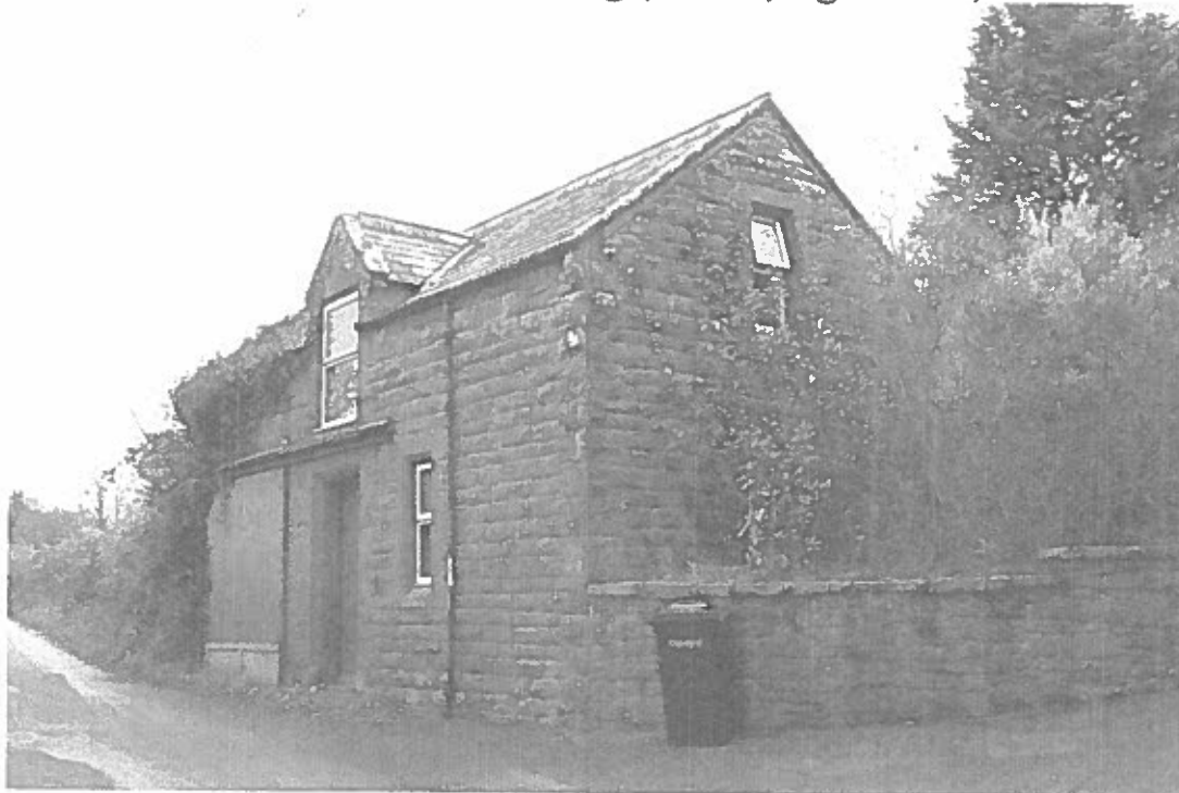
Coach House viewed from the northwest
