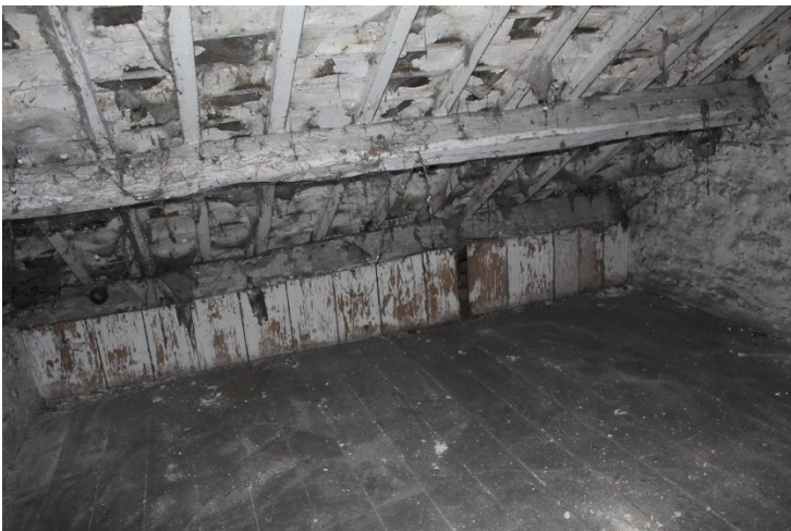
Roof void in the north Area illuminated from roof lights Cobwebbed Eaves boarded out
