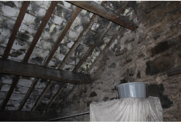
Roof void in the south Dark and cobwebbed Parge coating in poor condition Timber beams in good condition
