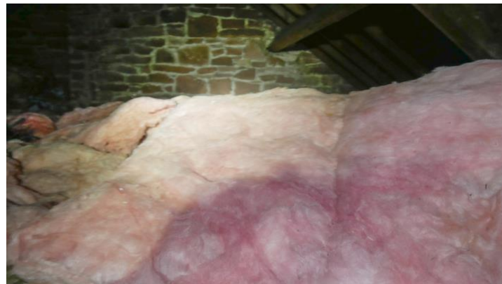
5. Most floor areas in roof space have rockwool type insulation which makes evidence searching effective
