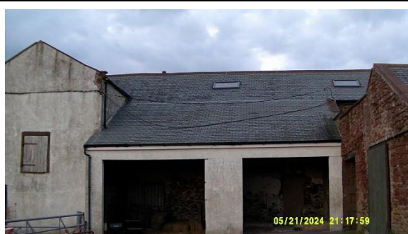
Photo 7: 21-05-24 Building 5 S4 survey start
