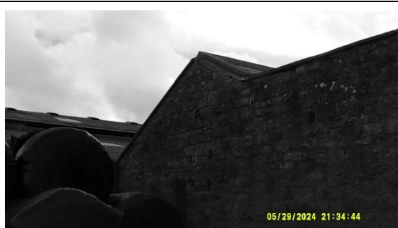
Photo 11: 29-05-24 Building 3 S3 survey start
