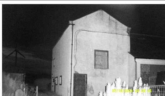
Photo 2: 10-07-24 Building 6 S6 survey end
