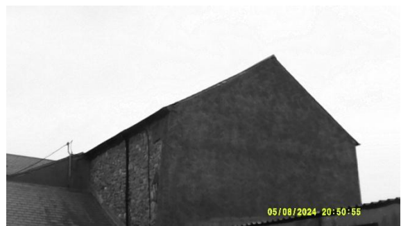
Photo 2: 08-05-24 Building 1 S2 survey start
