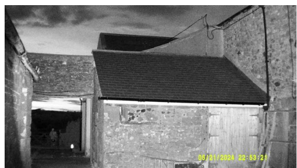
Photo 6: 21-05-24 Building 1 S2 survey end
