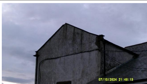
Photo 15: 10-07-24 Building 6 S4 survey start
