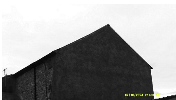
Photo 15: 10-07-24 Building 1 S2 survey start
