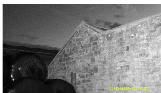
Photo 14: 29-05-24 Building 3 S3 survey end
