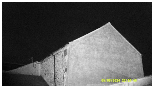
Photo 4: 08-05-24 Building 1 S2 survey end
