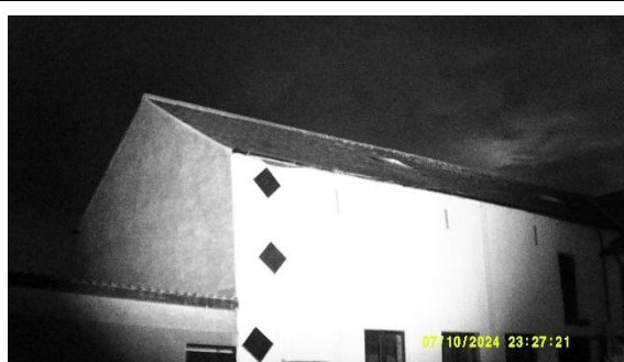
Photo 2: 10-07-24 Building 1 S1 survey end
