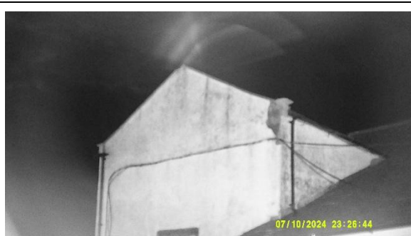
Photo 15: 10-07-24 Building 6 S4 survey end
