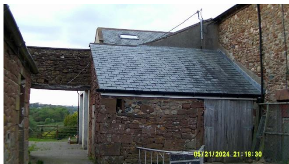
Photo 5: 21-05-24 Building 4 S2 survey start
