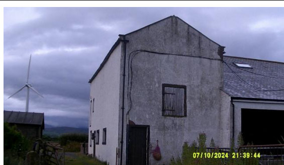
Photo 2: 10-07-24 Building 6 S6 survey start
