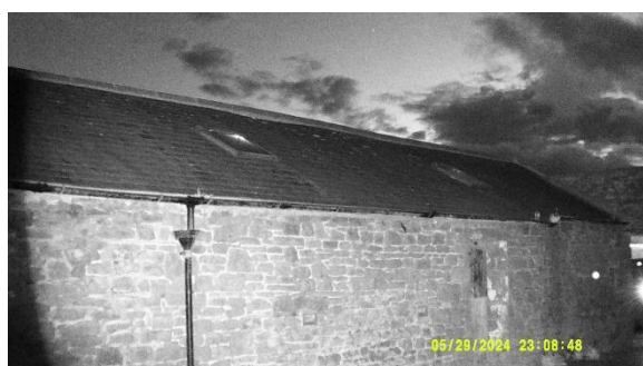
Photo 15: 29-05-24 Building 3 S2 survey end
