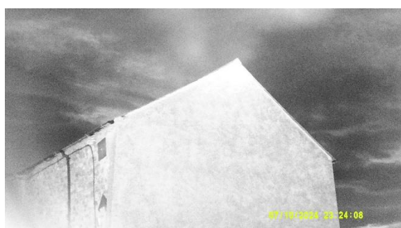
Photo 15: 10-07-24 Building 1 S2 survey end
