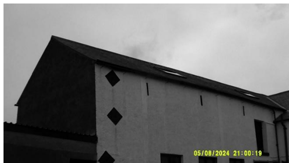
Photo 1: 08-05-24 Building 1 S1 survey start
