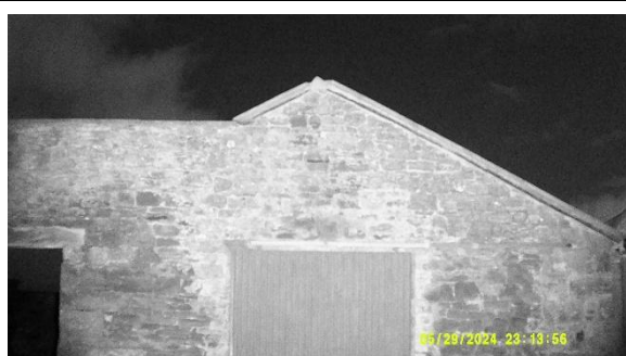
Photo 13: 29-05-24 Building 3 S5 survey end
