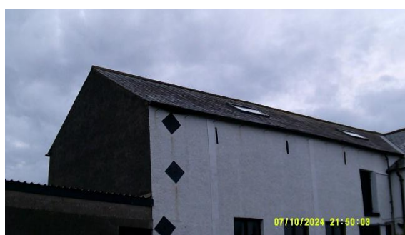
Photo 2: 10-07-24 Building 1 S1 survey start
