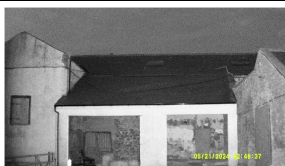
Photo 8: 21-05-24 Building 5 S4 survey end
