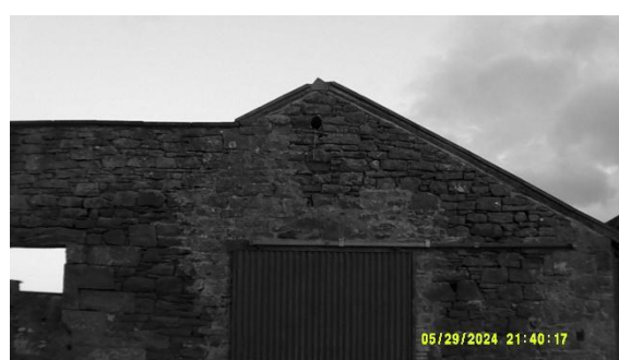
Photo 10: 29-05-24 Building 3 S5 survey start
