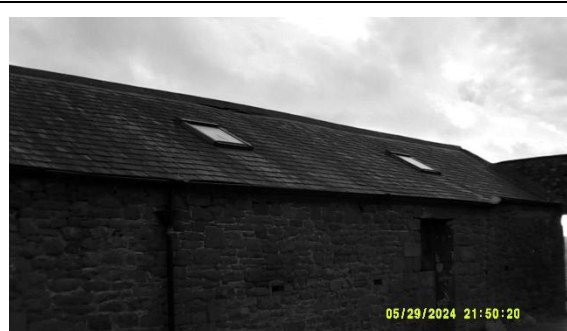
Photo 12: 29-05-24 Building 3 S2 survey start
