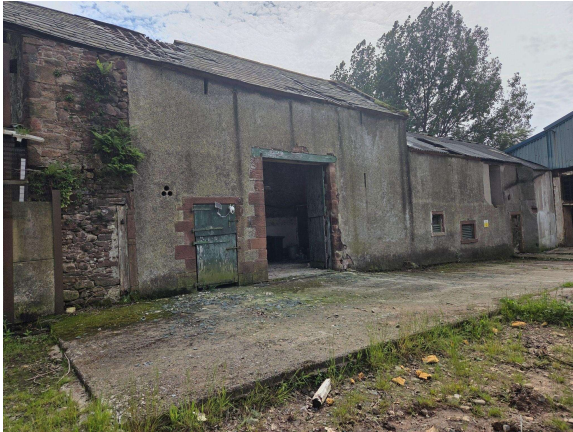
Photo above: External view of stone barn that is not due to be removed from the site. Building has two stories with the upper story being unstable for access.
