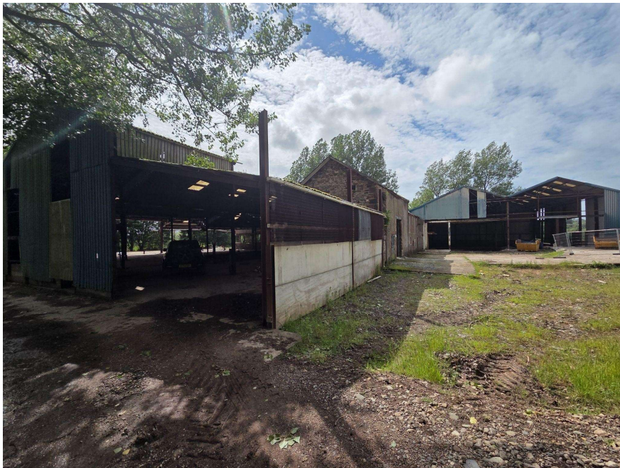
Image: Overview of survey barns (Left to right: Barn 1, Stone Build, Barn 2)
