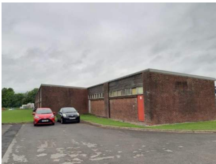
Photograph 1 – Eastern corner of Unit 15A-H on Leconfield Street
