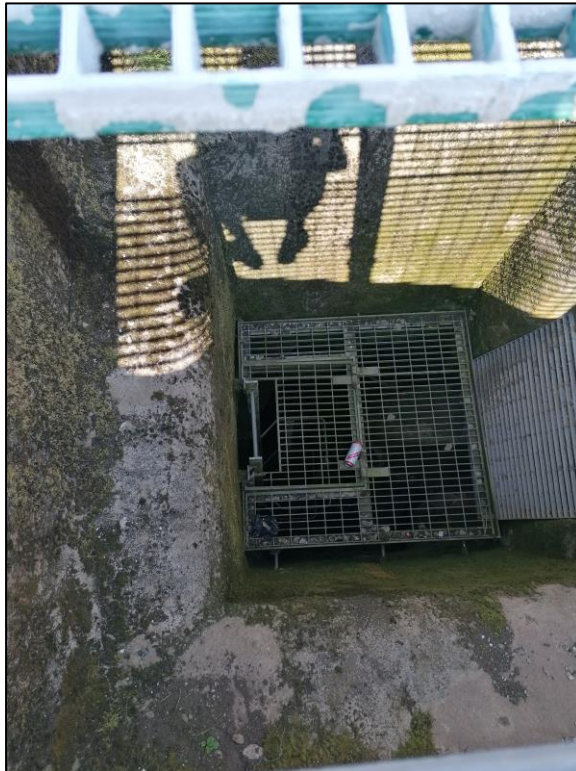
Photo 2 – Northern Discharge Pipe – Shaft (II)
