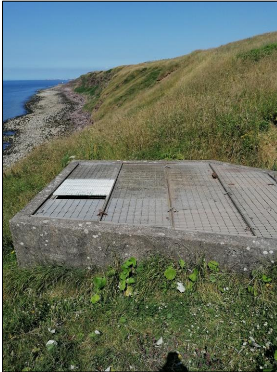
Photo 1 – Northern Discharge Pipe – Shaft (I)
