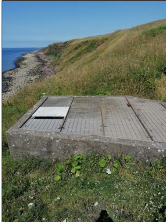
Photo 1 – Northern Discharge Pipe – Shaft (I)
