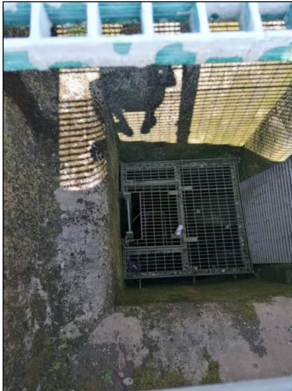
Photo 2 – Northern Discharge Pipe – Shaft (II)
