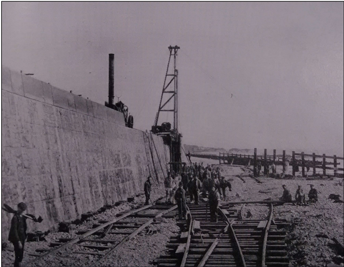
Plate 7: The Inner Barrier under construction (after Harris 1970)
