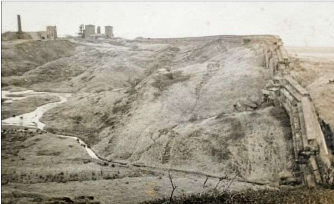
Plate 9: 'Top slicing' and the effect on the Inner Barrier, c. 1920 (Cumbria Image Bank ct12541)
