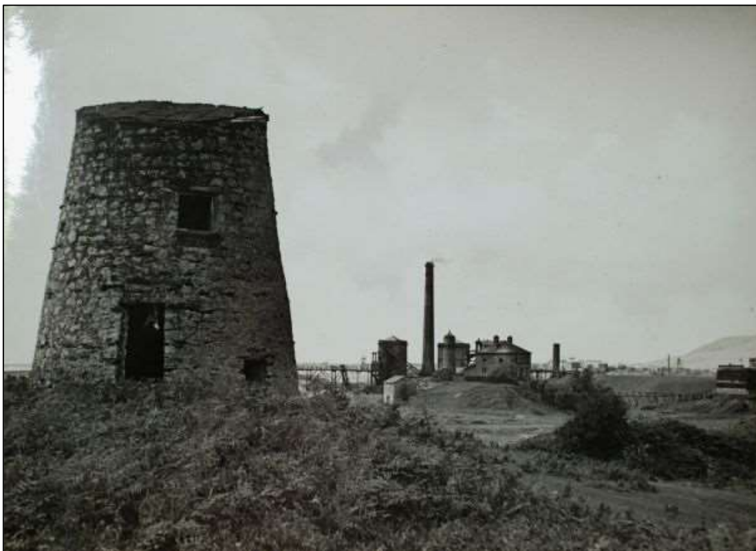
Plate 4: Derelict Windmill with mine workings (Cumbria Image Bank ct12499)
