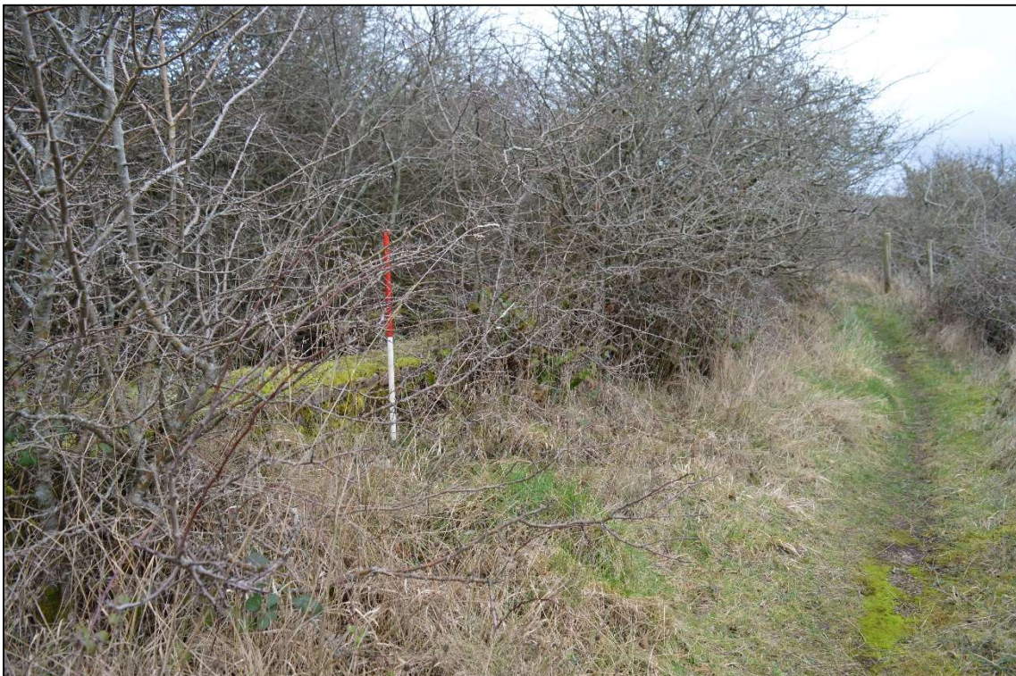
Plate 12: Structural remains of a bridge wall (WA058)
