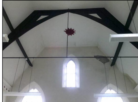
Figure 18. Roof truss, cross-bar and air vents
