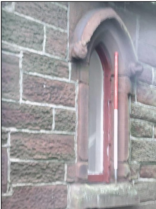
Figure 19. Gothic style window to porch
