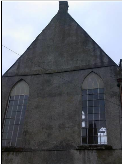
Figure 12. Upper west elevation
