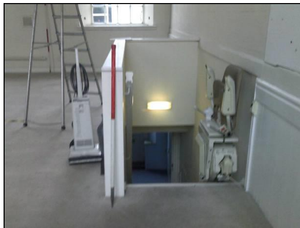
Figure 22. Stairs linking the floors
