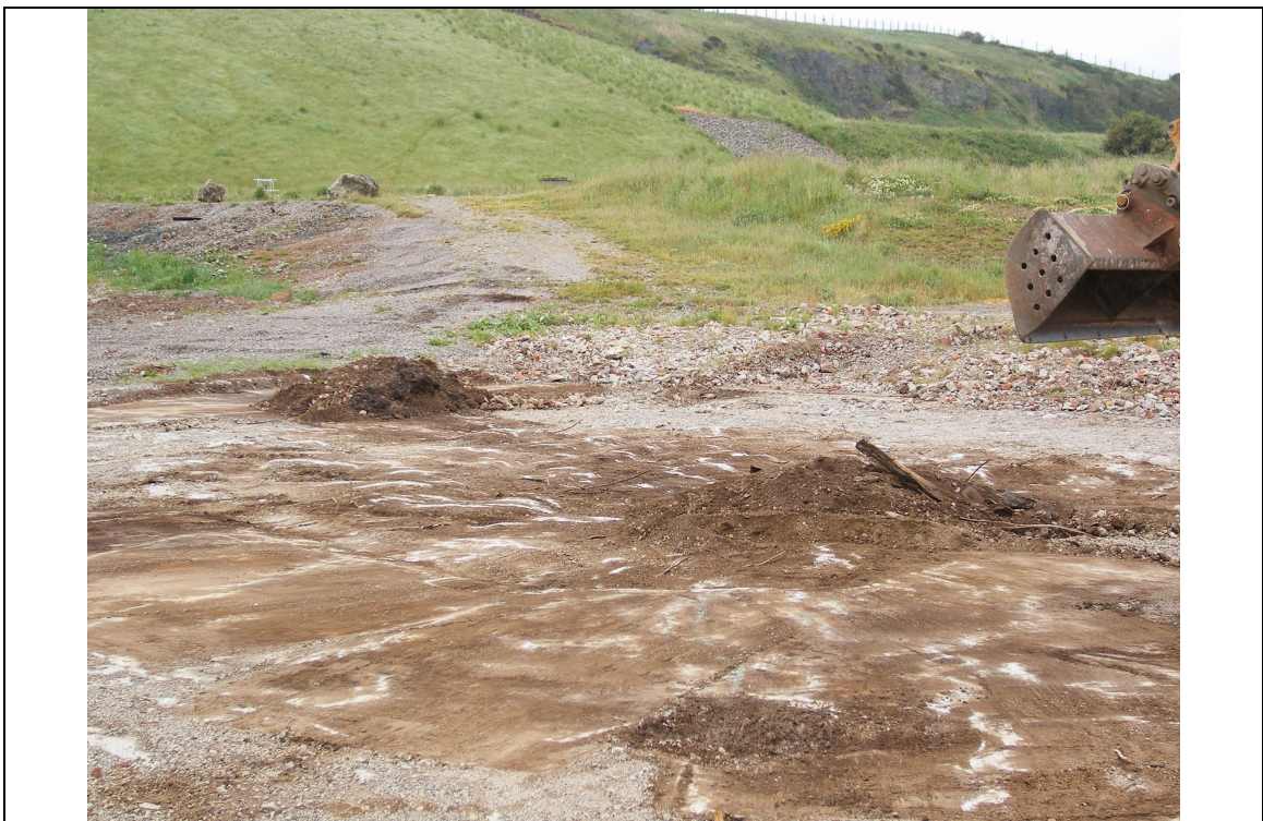
Photograph No: 4 CHP scrape in progress showing concrete hardstanding in good condition, June 08
