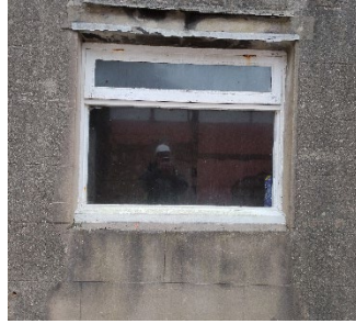
TOP OPENING MODERN TIMBER CASEMENT
