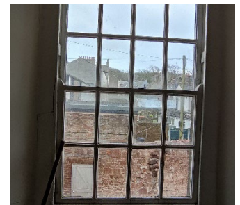
MODERN 8/8 BOX SASH NO SHUTTERS
