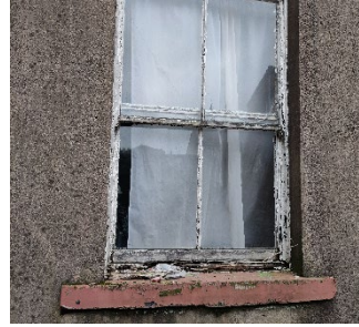
MODERN 2/2 BOX SASH FRAME - DECAYED
