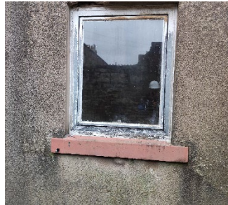
MODERN TIMBER CASEMENT WINDOW
