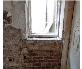
WINDOW OPENING TO BE RESTORED AS DOOR – INT VIEW
