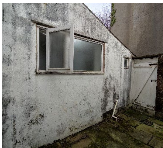
MODERN TIMBER CASEMENT WINDOW
