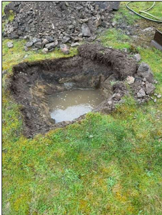
Figure 2: Photo of the trial hole taken at 14:00
