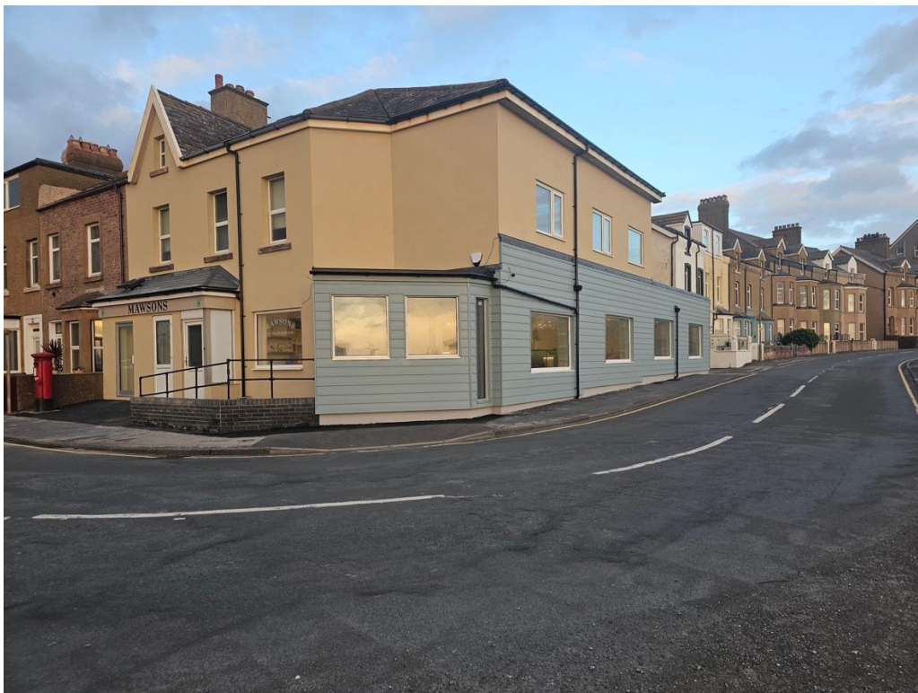
Post Development photograph, due to cracking the external leaf has been taken down and re-built. New doorway shown to bakery – compliant disabled ramp installed for level access and storm porch to protect from storms / sea on opposite side of carriageway.
