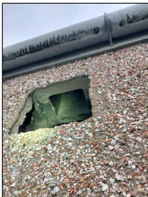
Photograph 9: Hole leading into cavity of breeze block (also shown in photograph 8).
