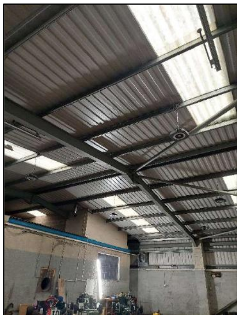
Photograph 9: Internal of building reference B with internal office at ground level.
