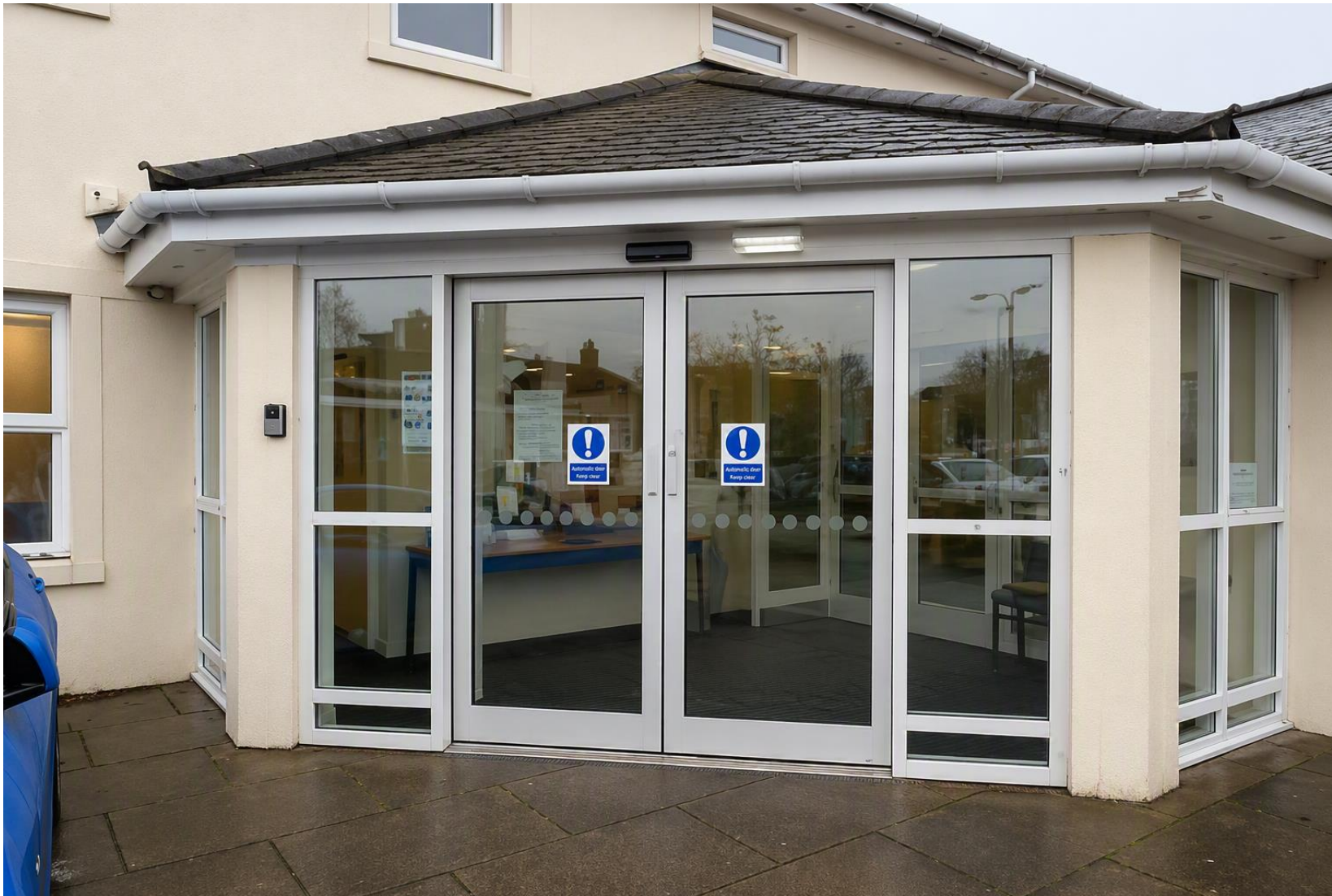
External View – Provided buy window installer of replacement doors.
