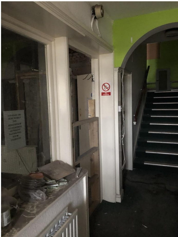
Image 1 - Internal View towards main staircase from new vestibule, proposed Apartment 1 to left hand side – modern glazed screen forming the original reception counter for the previous owners.
