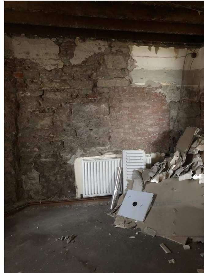
Image 4 - Rear wall in the new café, a former opening in the rear wall indicated (not visible externally) and overlapped by the current external staircase. This window is in the location of the new café toilet and will not be visible internally when works are complete.
