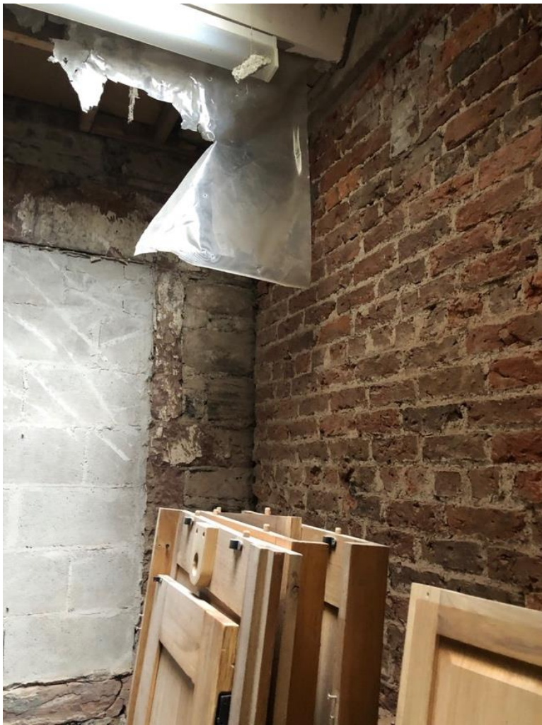
Image 7 – Infilled window as Image 6, the right hand flank wall forms the rear stairwell wall to the property which is paint finished on the upper level of the stairwell
