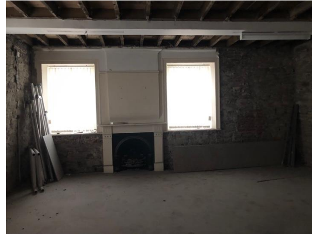
Image 12 – View internally in Apartment 3 to gable wall with fire place centrally between windows. Current fireplace and surround to be retained in situ -see image 13
