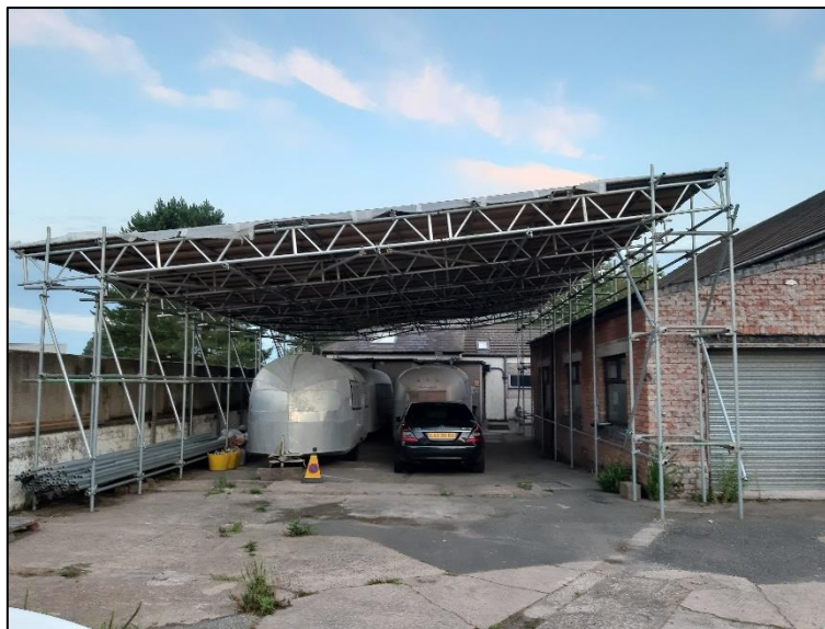
Photograph 1 – Showing external scaffold with a plywood roof.
