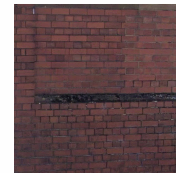
Sample swatch of existing brickwork to be retained.
