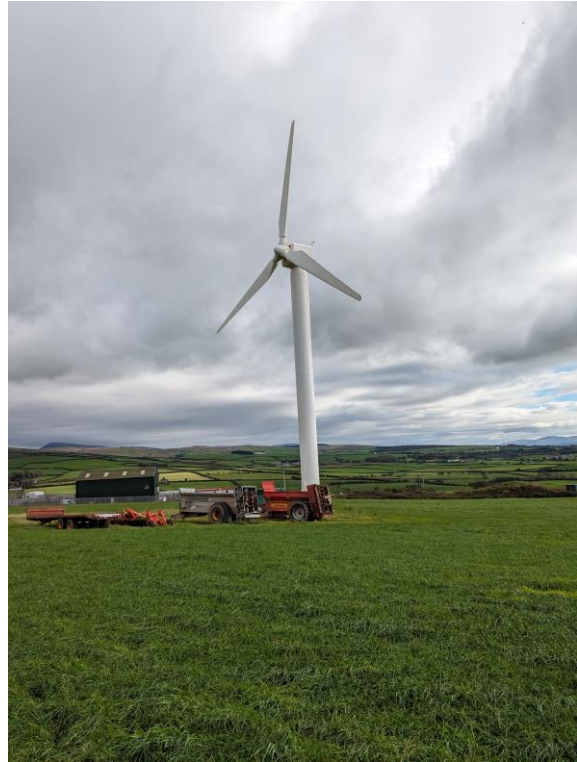
Photo 7: T1, existing turbine.
