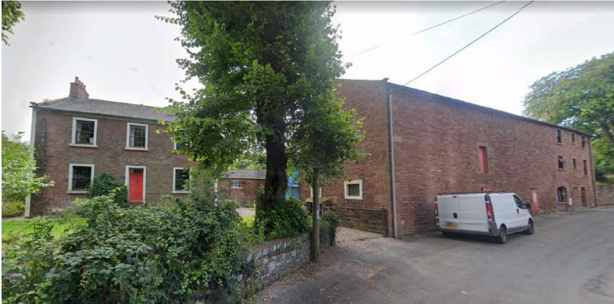
Plate 16. NHLE 1086616 Grade II House and NHLE 1359643 Grade II Barn facing east.
