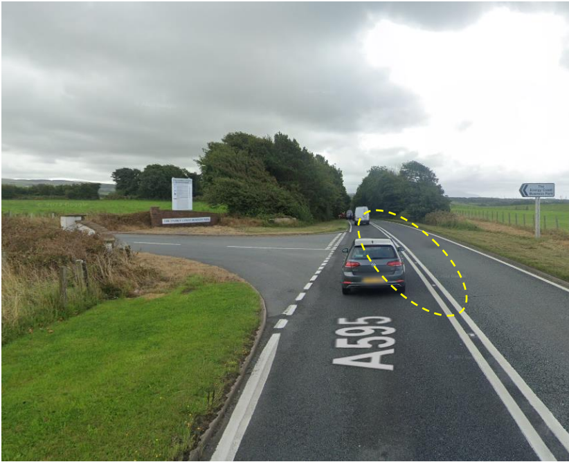
Plate 6: Photograph showing A595 junction/minor public road with identified oversail point
