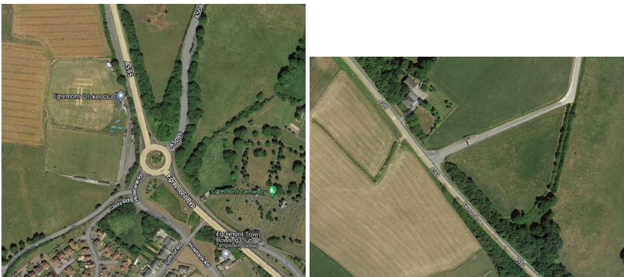
Plate 4: A595 Egremont Roundabout (left) and A595 Entrance to Business Park (right)
