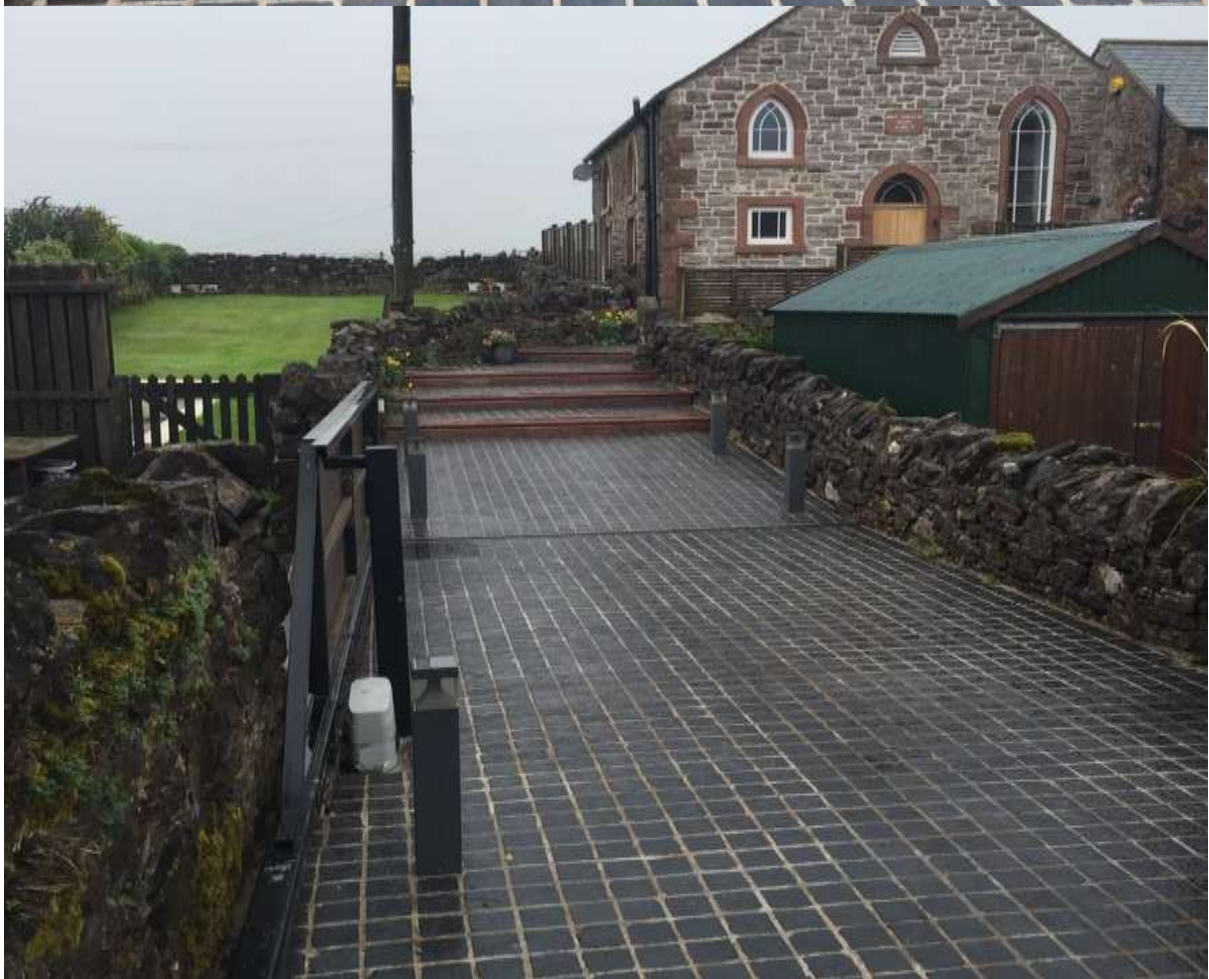
Set Paving (as existing) Looking westward to the Front elevation of Kirkland Chapel (east elevation)
