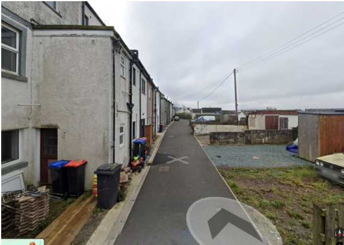
Non-adopted road to rear of 3 Lake View (looking southward)
