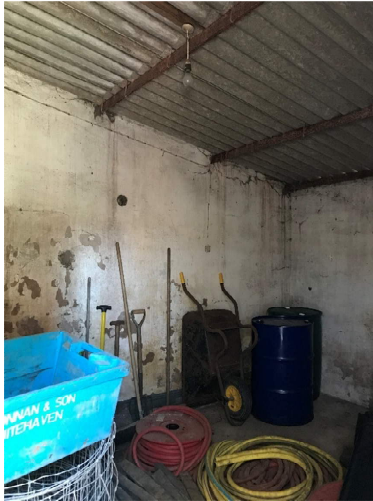
Figure 3.6 – Water staining and cracking to internal wall
