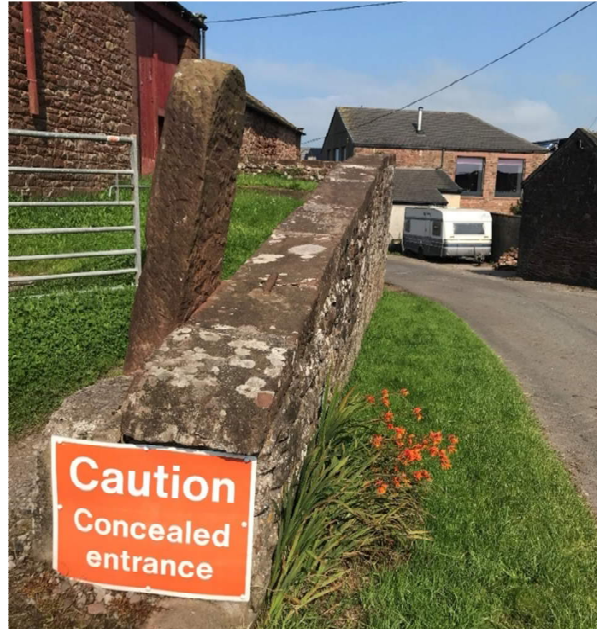
Figure 3.0 – Lean in retaining wall to Barn One
