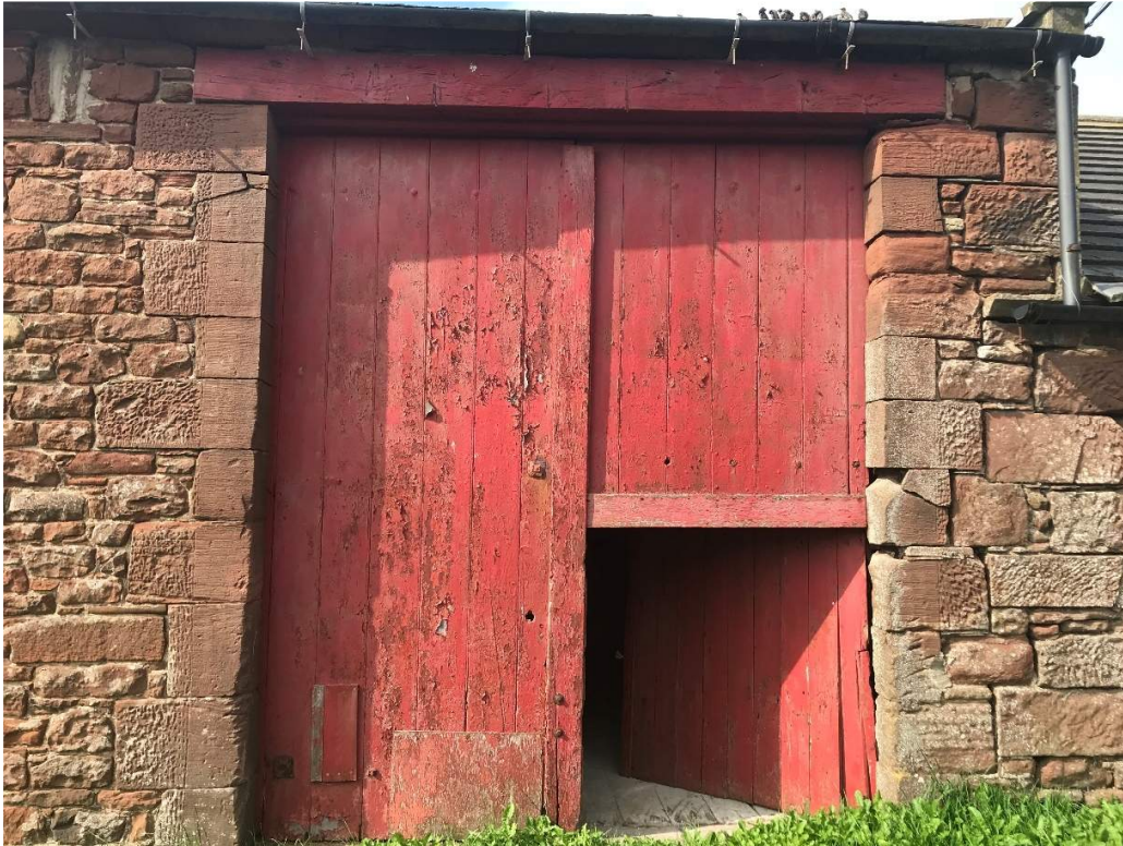
Figure 3.10 – Broken stones around door
