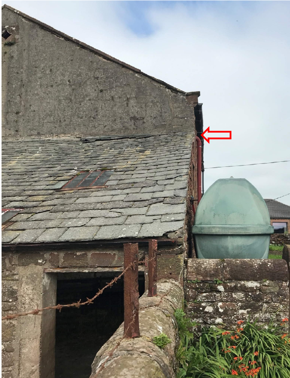
Figure 3.9 – Inwards dish in front wall
