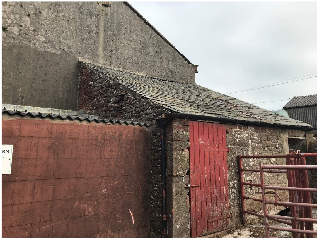
Figure 3.7 – Dip in roof of stone lean to extension
