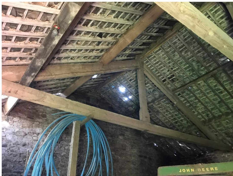
Figure 3.11 – Barn One roof trusses
