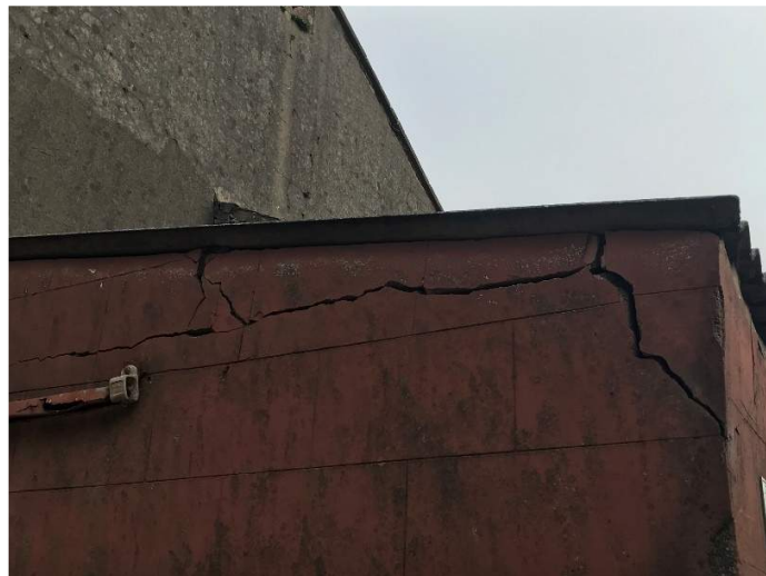
Figure 3.5 – Cracking at purlin bearings
