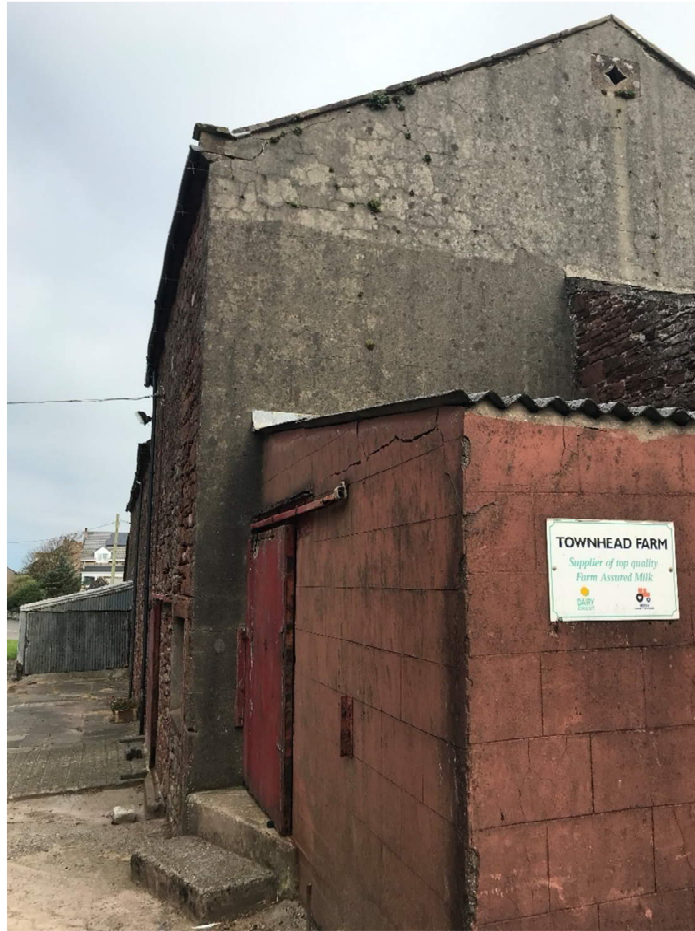
Figure 3.4 – Loose stones at eaves and cracking to extension
