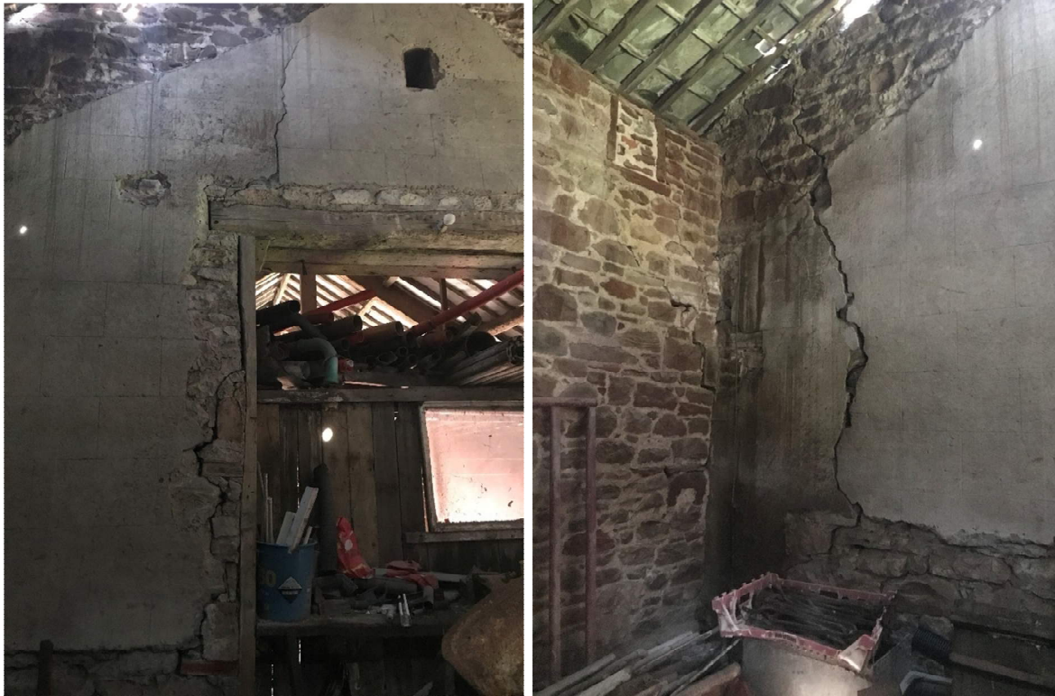
Figure 3.12 – Cracking in internal wall
