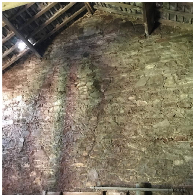
Figure 3.13 – Vertical crack in gable
