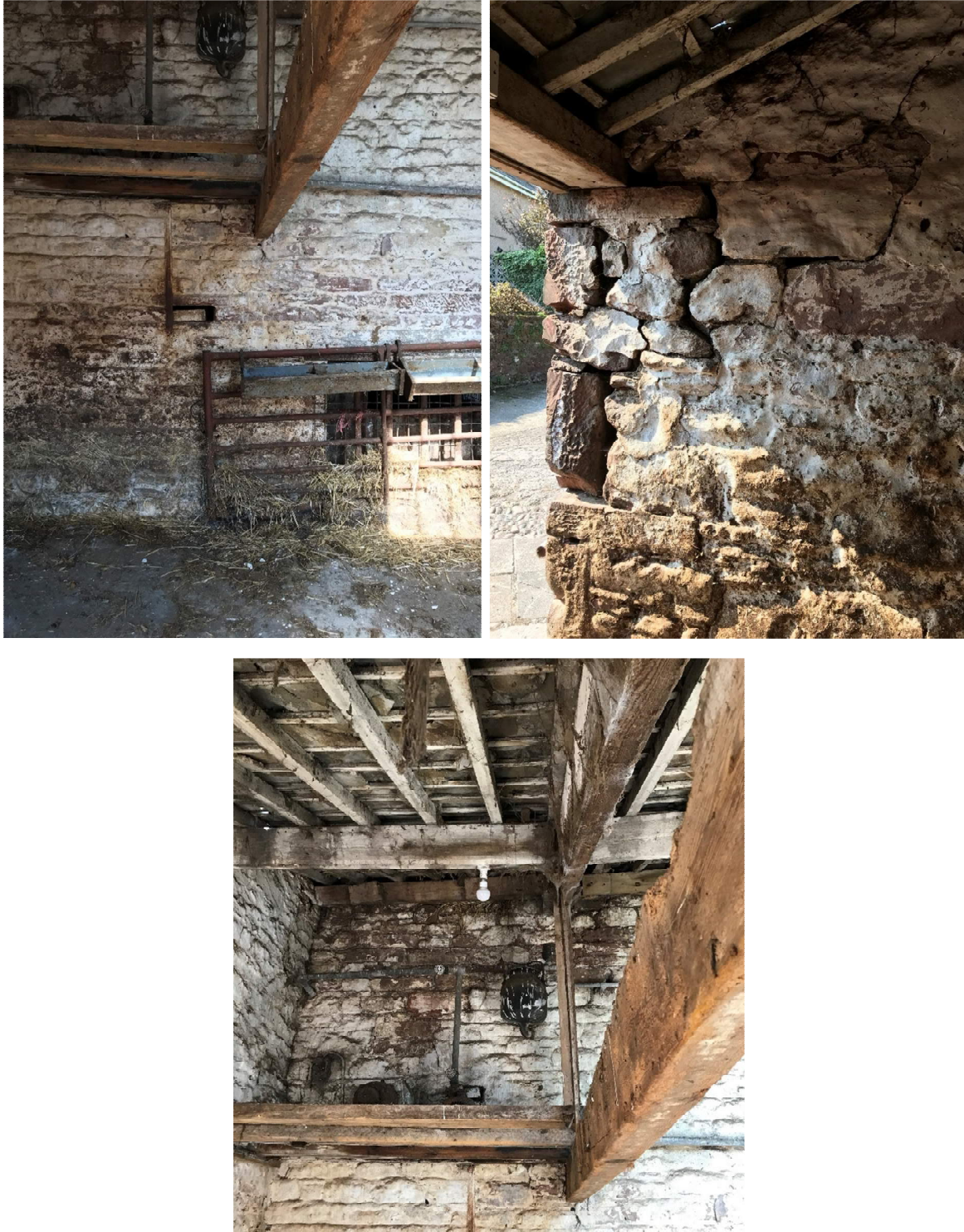
Figure 3.8 – Cracking at truss bearing, loose stone by door and dip in purlin
