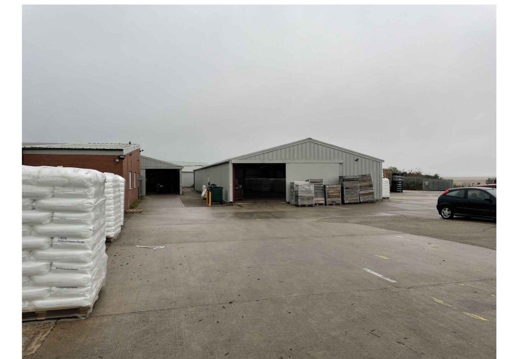
PHOTO OF EX. WAREHOUSE FROM SOUTH WEST
