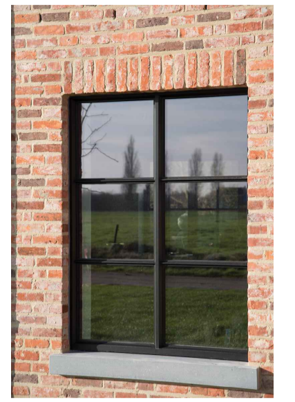
Example of aluminium windows - Slimline profiles e.g. Reynears SL38 Colour - Grey
