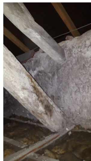
Figure 5: Part of existing truss with new rafters and felt over.
