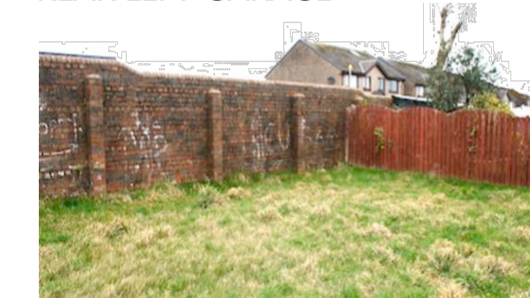
WALL TO no.179( FENCE
