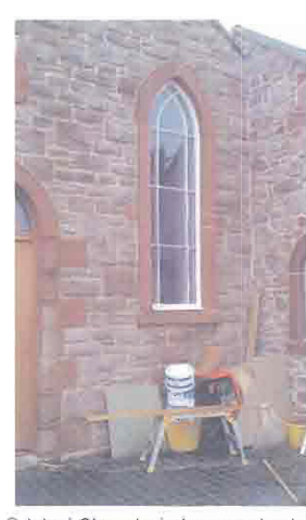
Original Chapel window opening left unaltered and new purpose made replacement window manufactured to suit opening
