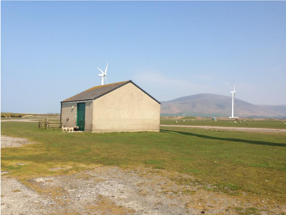
Haverigg III substation
