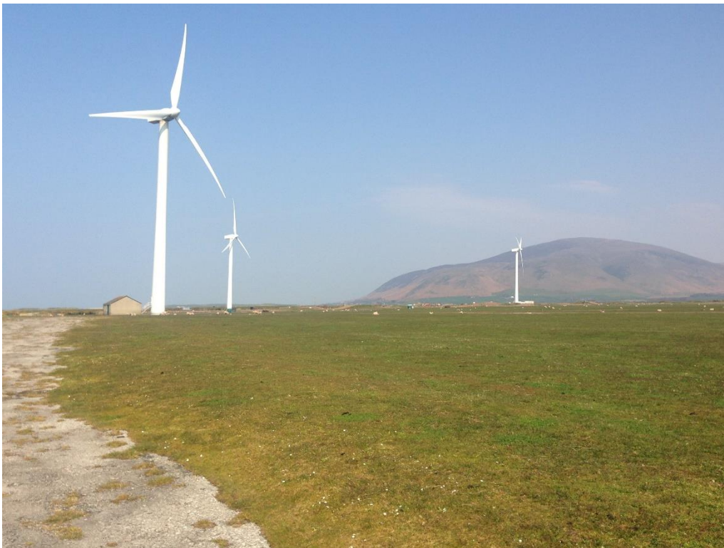
Turbines at Haverigg III
