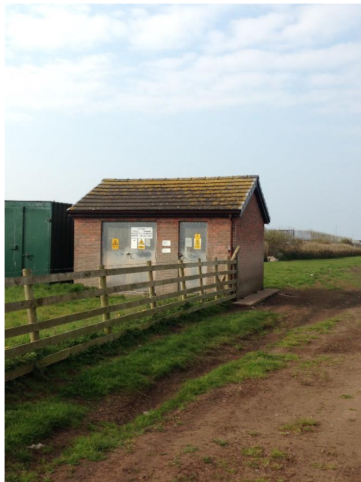
Haverigg II substation adjacent to entrance from North Lane
