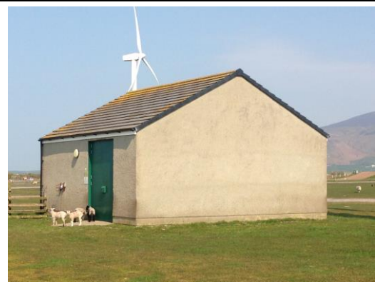
Photograph 8: Substation with Haverigg III.
