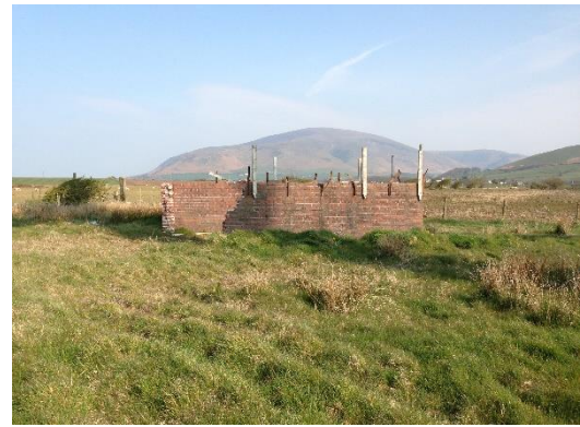
Photograph 8: Half built structure in motocross area.
