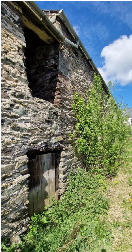
Photo 11 - east Elevation of Barn 3 - Lateral Movement
