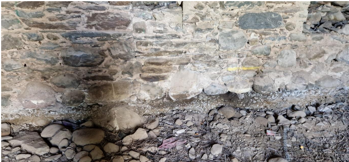
Photo 5 - Barn 3 - Excavations Below Foundation Stones
