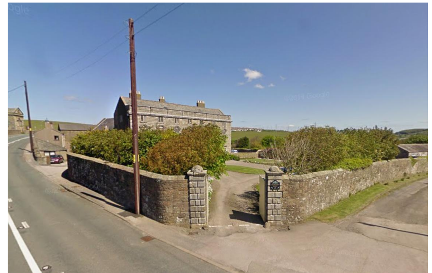
Entrance Walls & Gate Piers to Moresby Hall
