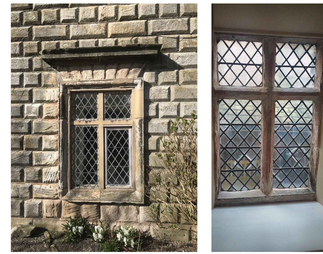
Photographs of typical external & internal window arrangements to front elevation.
