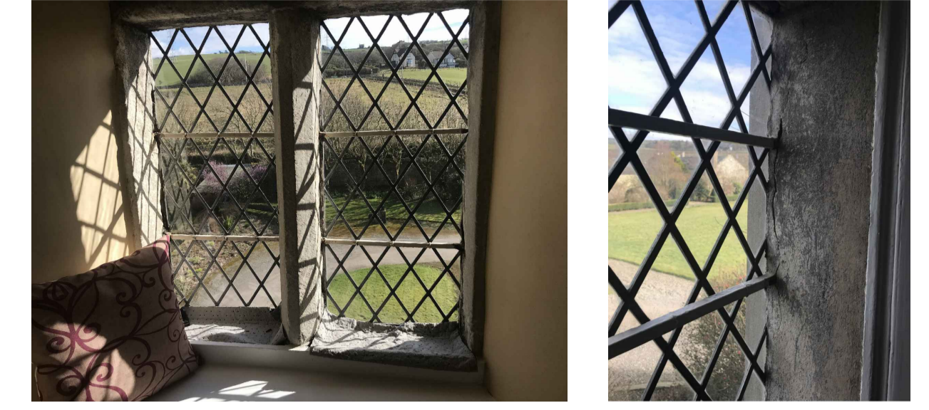
Photographs of typical ironwork to existing windows.
