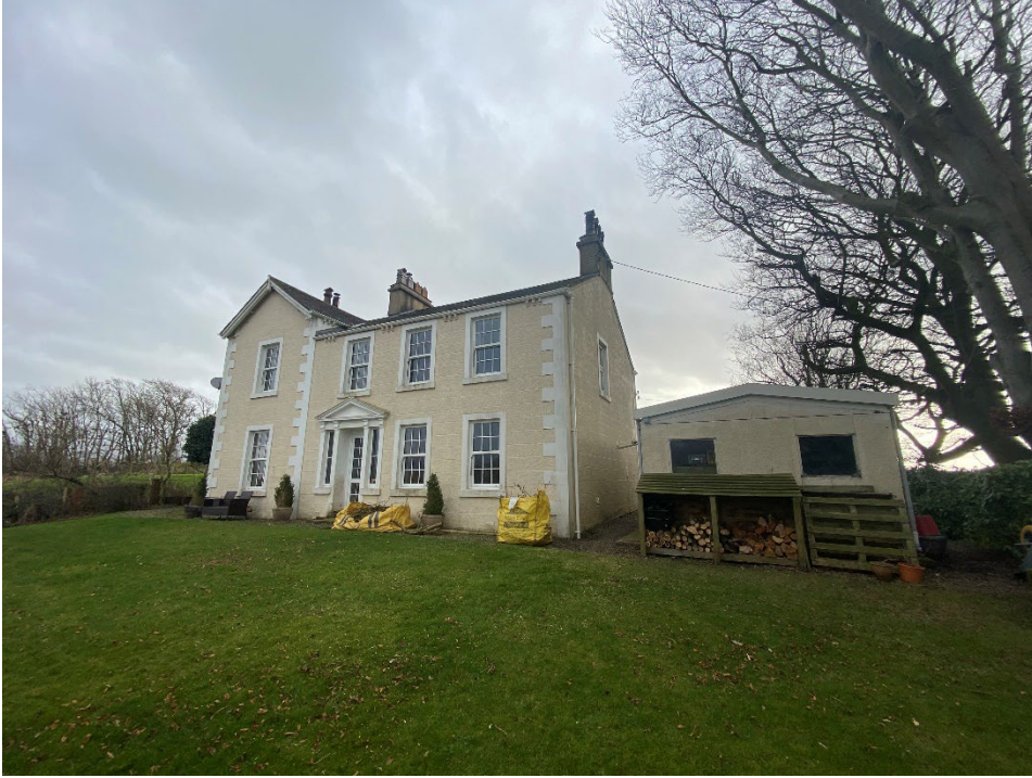
View of the North elevation of the existing dwelling.
