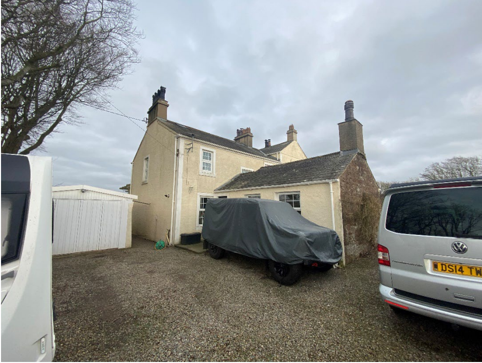
View of the West elevation of the existing dwelling.
