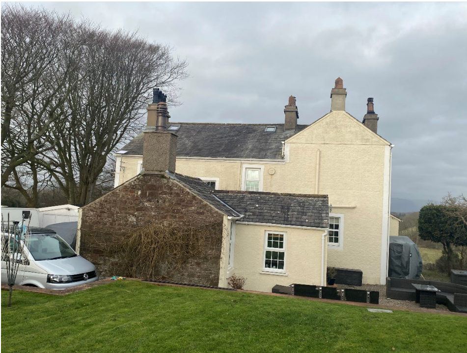
View of the South elevation of the existing dwelling.
