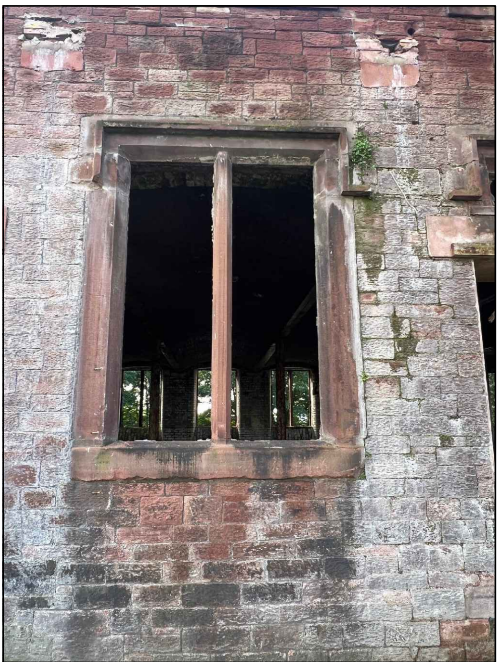
PHOTO OF TYPICAL WINDOW EXTERNALLY SHOWING STONE COLUMN.
