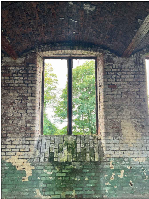
PHOTO OF TYPICAL WINDOW INTERNALLY SHOWING A METAL COLUMN
