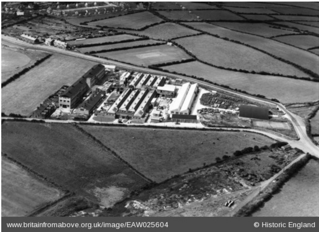
1 The Tannery complex as recorded in 1949, at the peak of its production capacity. Office building and entrance in the foreground.
