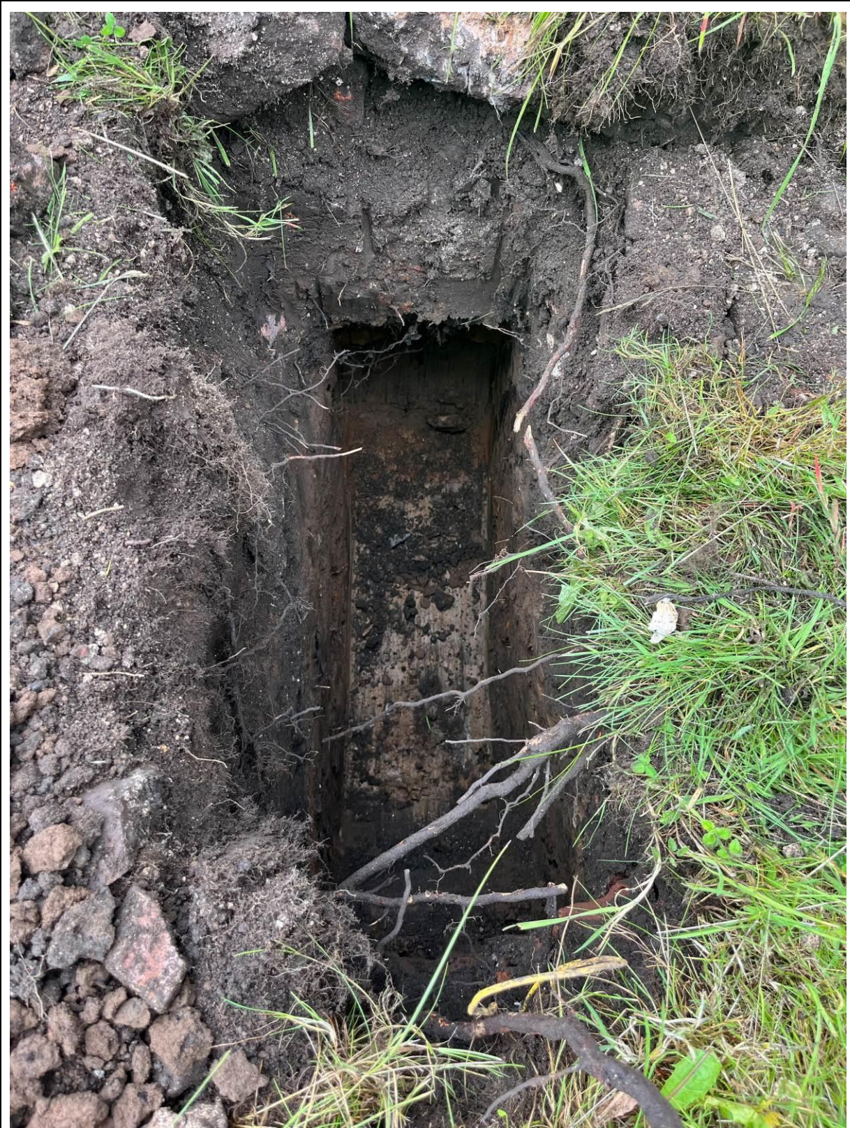
Photo 5: SA02 on completion
