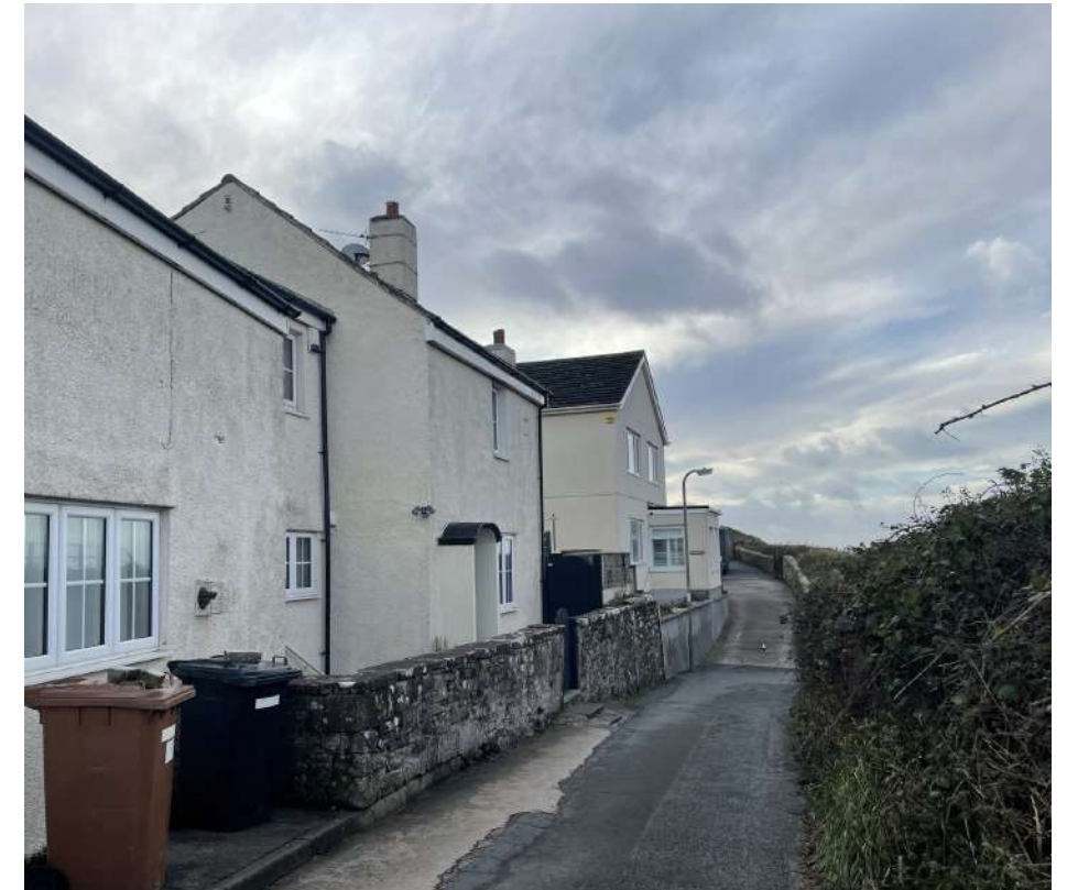
View South from Marsh House towards Stoney Croft
