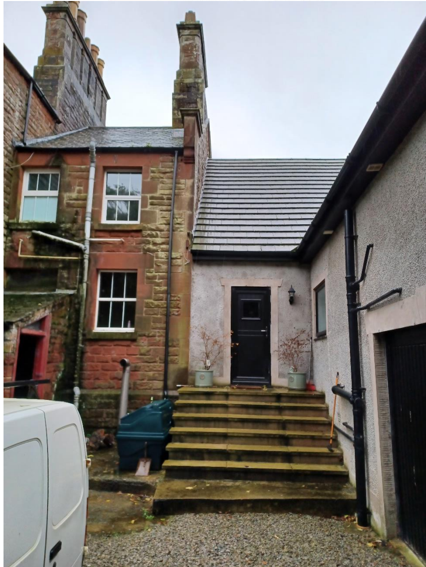
Photograph 2 – existing access steps. Main Rothersyke House to left. Proposals for the extension provide a wider set of steps, leaving space for a lifting device, landing area and safe balustrading.
