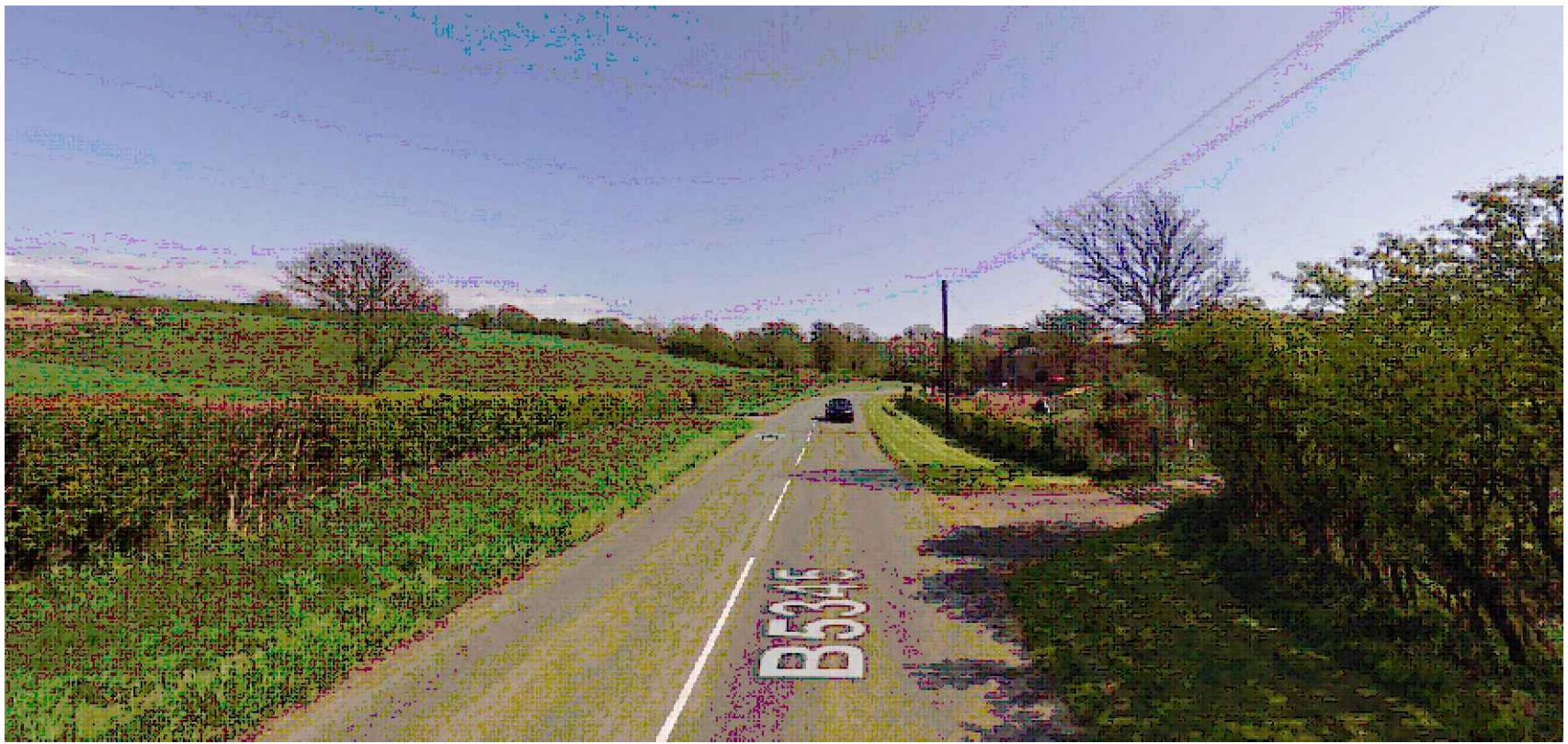
P2 - Visibility of access road facing Southeast.
