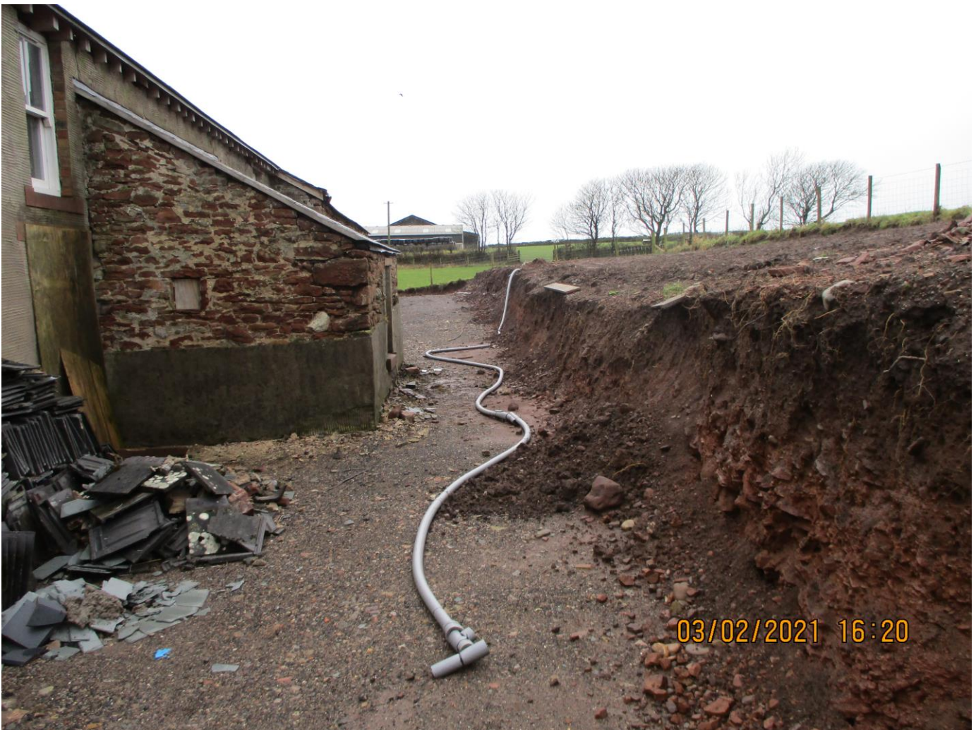
Photograph showing the reduced level excavations along the rear of the property.
