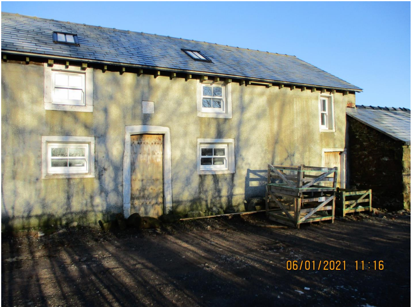
Photograph of the front elevation showing the existing farmhouse render finish, new roof slates, eaves level and detail and replacement windows.
