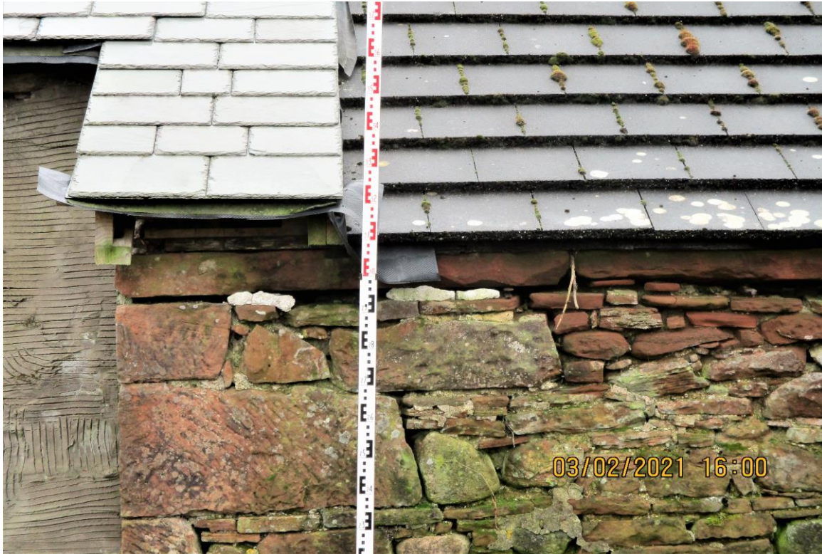
Detail of the rear barn wall showing the poor quality small weathered stone pieces.
