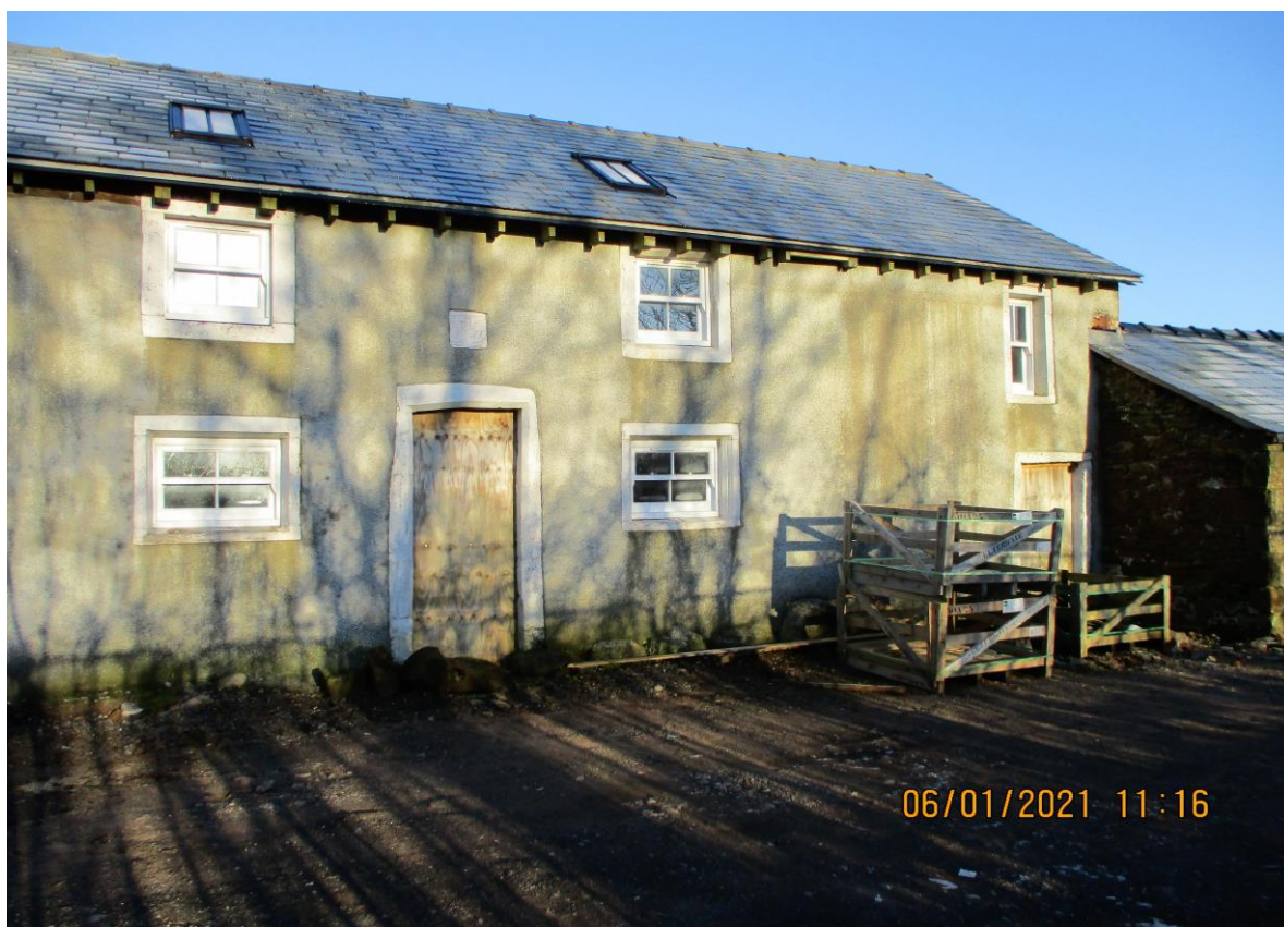
Photograph of the front elevation showing the existing farmhouse render finish, new roof slates, eaves level and detail and replacement windows.
