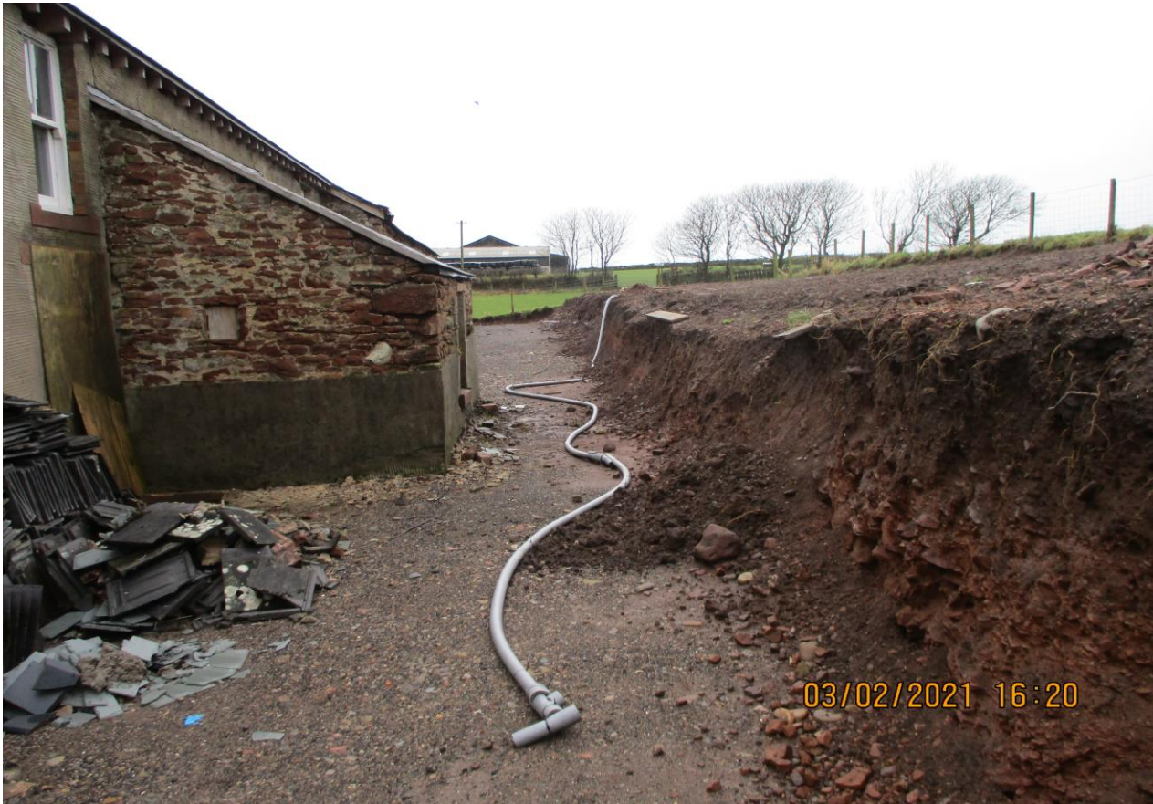
Photograph showing the reduced level excavations along the rear of the property.
