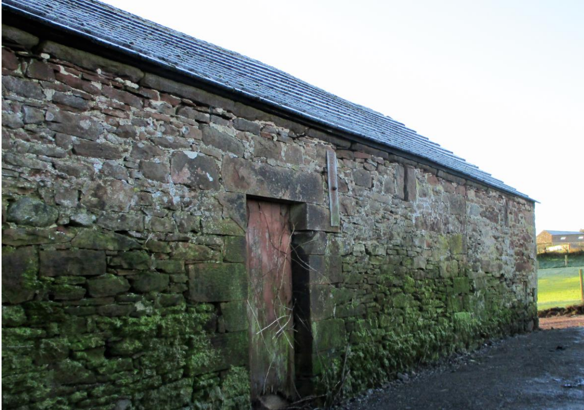
Photograph of the existing rear barn wall showing the effect of the weathering, the structural support plate will be removed when the front wall is re-constructed.
