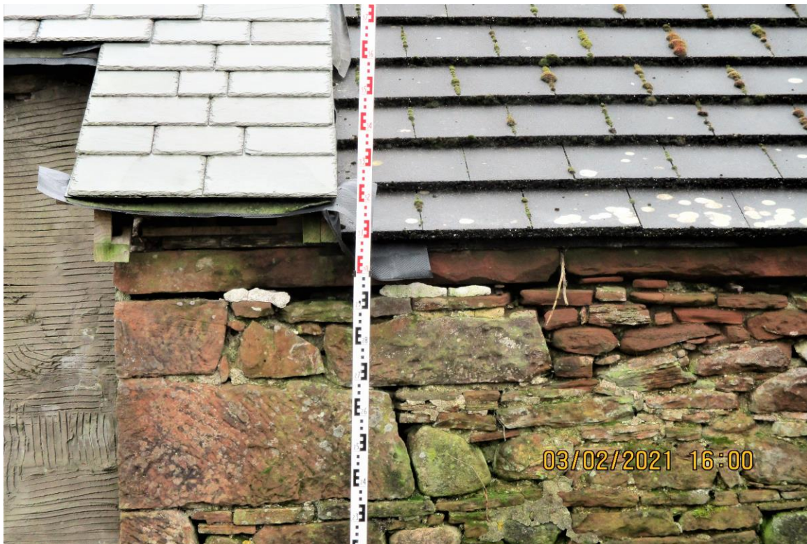
Detail of the rear barn wall showing the poor quality small weathered stone pieces and also showing the junction of the different roof level and finish, the barn will be completed to match the left side dwelling roof, all as the originally consented details with the proposed render to match the dwelling.
