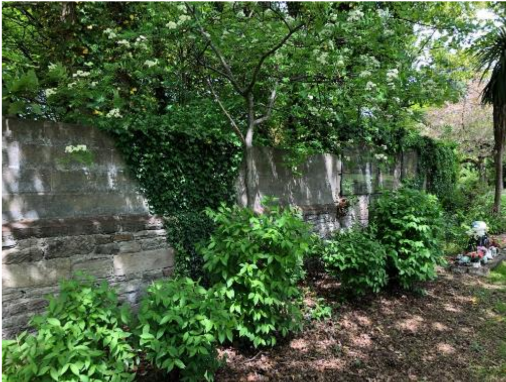
Figure 37 – Existing boundary wall, photographs taken from the neighbouring site, June 2022.
