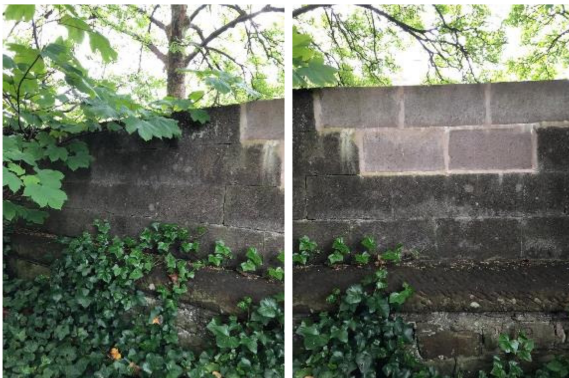
Figure 35 & 36 – Existing boundary wall, photographs taken inside the site, June 2022.
